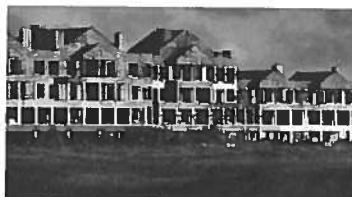
Condo project on hold in Galveston.
