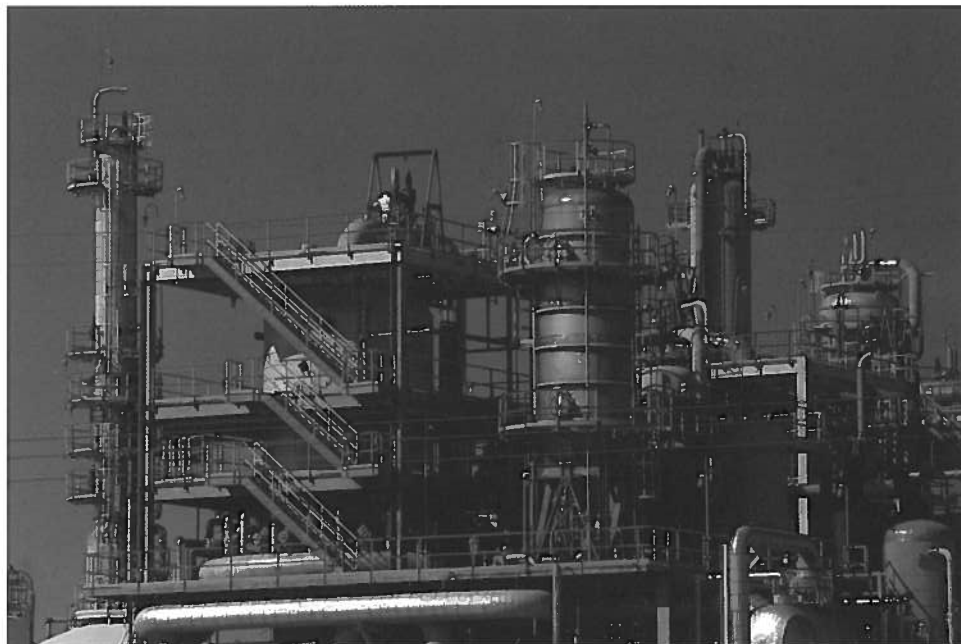
Formosa's original plant has been subjected to unprecedented state and federal fines for hazardous waste releases.
