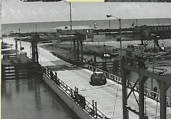
Sargent Beach, littered with wooden debris, appears sandy at first glance (left), but in reality is quite muddy. A simple summer shower can result in huge chunks of beach washing away (right). Below, the drawbridge over the Gulf Intracoastal Waterway is a mere stone's throw from the Gulf of Mexico these days. In some areas the two bodies of water are less than 300 yards apart.
