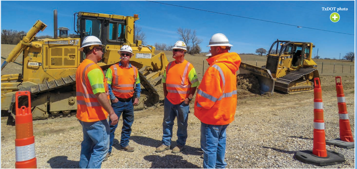
(l to r) Brownwood District Safety Officer Rex Miller, Fleet SWOT Specialist Luther Knight and Equipment Operators Mark Ogden and David Gillespie from the Waco District discuss creating firebreaks.
