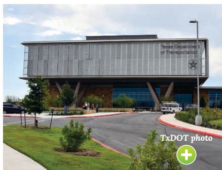
The Stassney Campus, the new home for more than 30 TxDOT divisions, opened in Austin in May.
