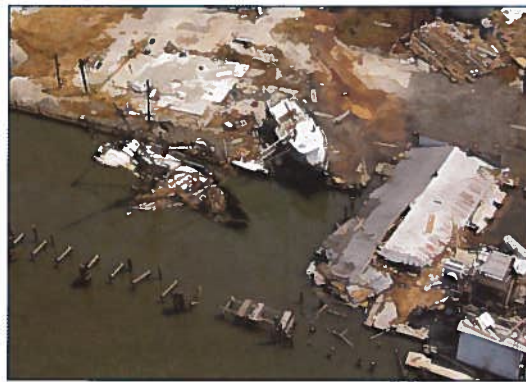
Grand Isle, La., after Hurricane Katrina.
