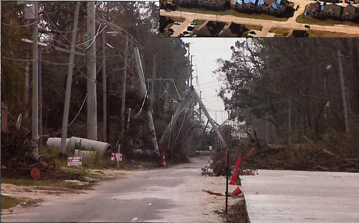
Downed power lines and fallen utility poles on Lake Street in Lake Charles.
