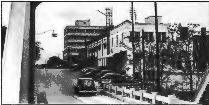
A West Texas Auto Company car crosses the "old" Kerrville bridge headed toward the Sid Peterson Memorial Hospital in the background and downtown. The hospital was under construction at the time.
