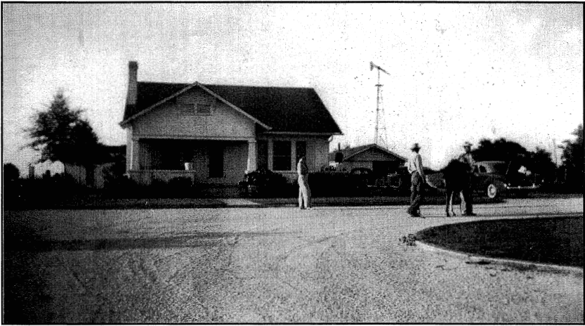
Above: The Diamond Bar Ranch house. It was a Peterson "home on the range" before Hal and Charlie bought Camp Eagle.
