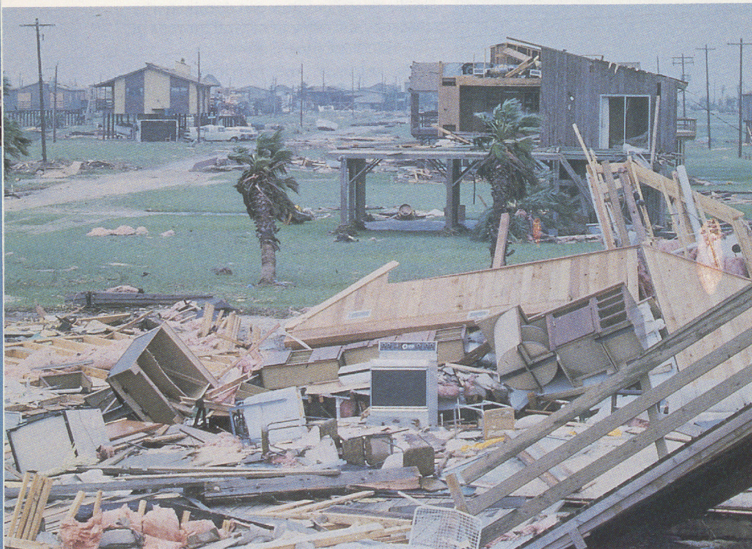
In Alicia's aftermath, it looked as though a giant bulldozer had been at work. Many of the homes in the area had been placed on pilings that did not hold when the structures were undermined by the storm surge or toppled over by heavy winds. Alicia was the costliest hurricane in Texas history, causing damages worth $2 billion to $3 billion.
