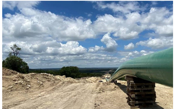
Pipeline construction in the Hill Country
