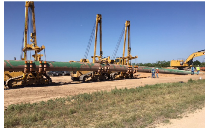
Pipeline construction in the Hill Country
