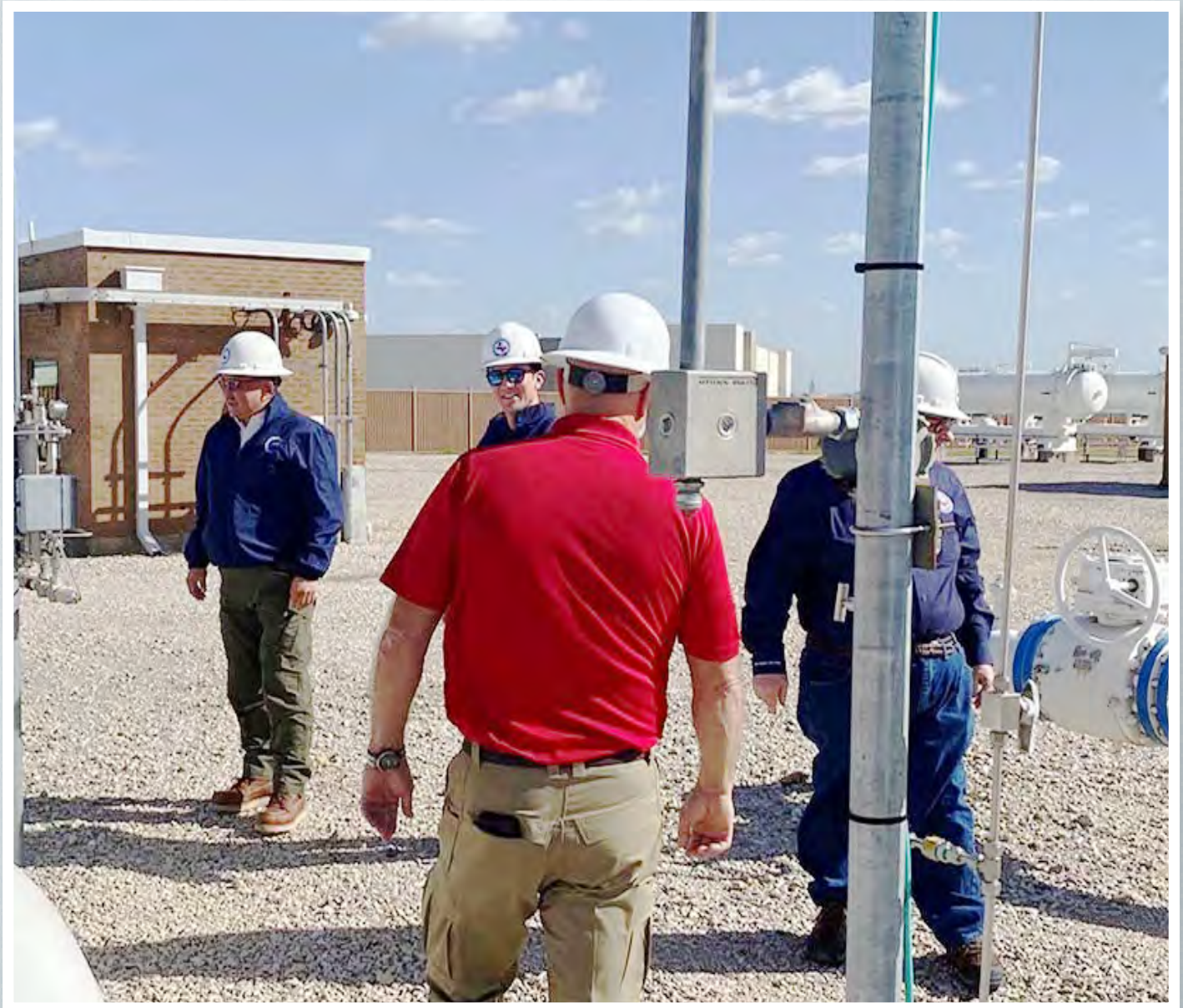
RRC leaders visit an underground gas storage and pipeline serving the Dallas/Fort Worth Metroplex. RRC has completed more than 1,000 site visits checking on the winter preparedness of natural gas infrastructure
