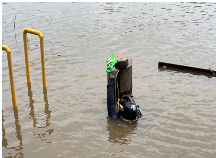
Diver working on surface casing
