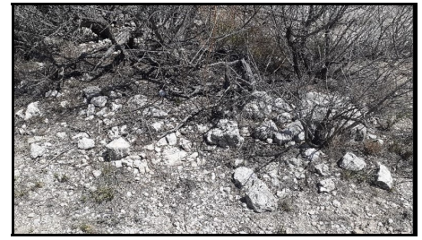
Figure 22. Constructed wall for the stone guard post platform.
