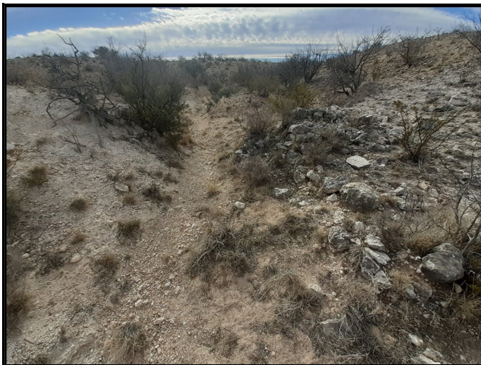
Figure 10. Remnants of Dam #1.
