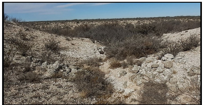
Figure 11. Remnants of Dam #2.
