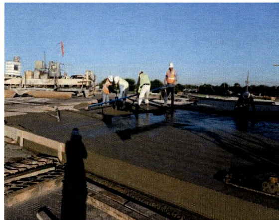
Figure 4.53 Concrete placement on the AL
