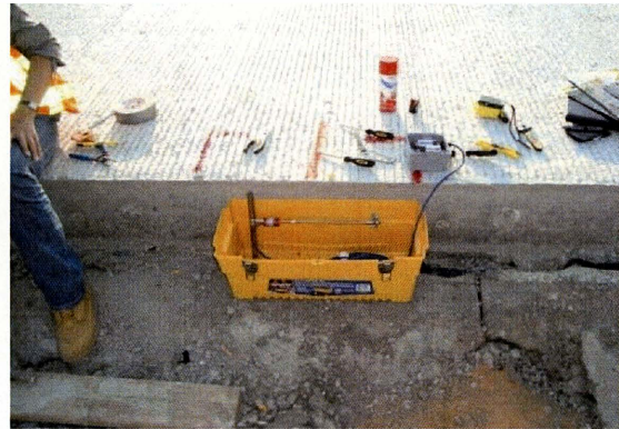
Figure 4.25 Installation of the crackmeter with protection box
