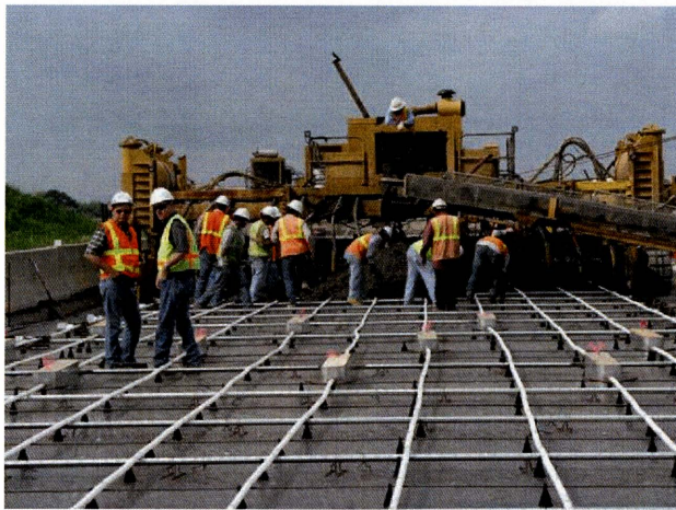
Figure 4.58 Pouring of concrete
