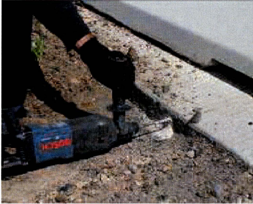
Figure 4.1 Drilling of transverse hole to install a groutable anchor
