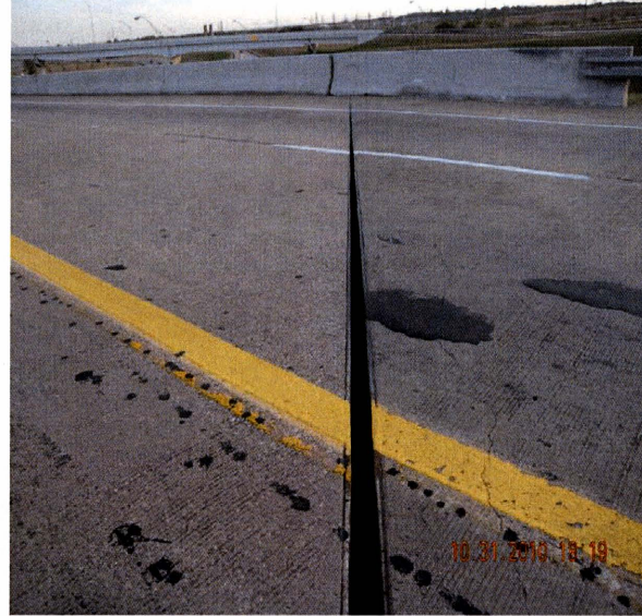
Figure 2.12 Variations in armor joint width
