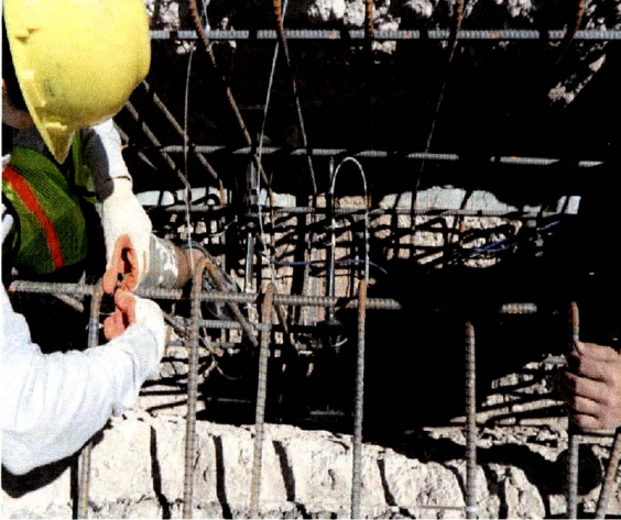
Figure 4.50 Installation of jackout pressure cells
