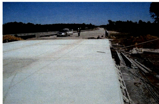
Figure 4.27 Pavement construction completed
