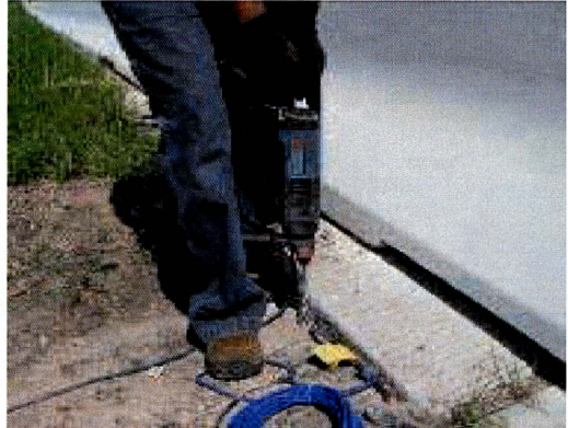
Figure 4.2 Drilling of a vertical hole to install invar
