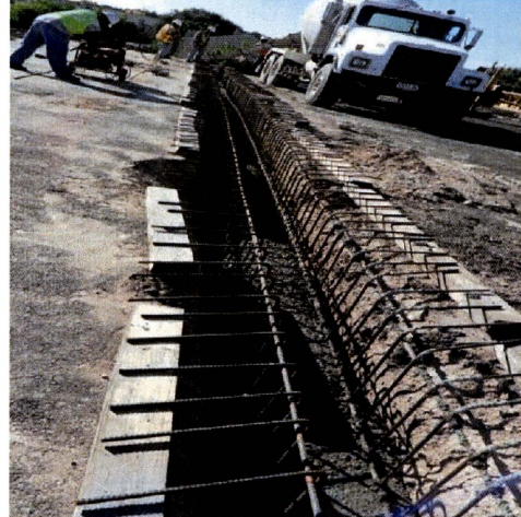
Figure 4.51 Concrete pouring in the lugs
