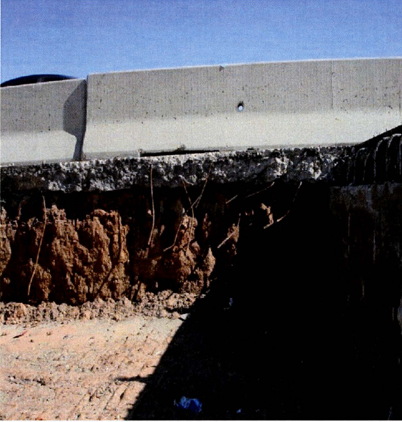
Figure 2.19 Bridge embankment and abutment
