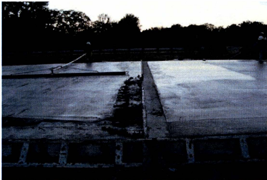
Figure 4.24 WF system placed
