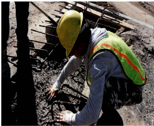
Figure 4.52 Covering the gages with concrete
