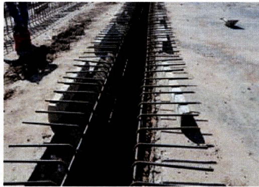
Figure 4.46 Cage tied and placed in the excavated area
