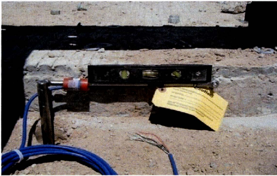
Figure 4.14 Installation of the crackmeter
