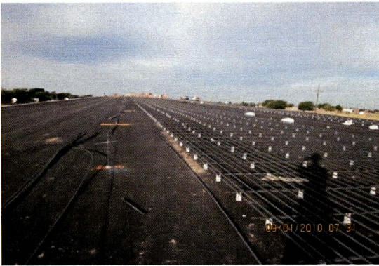
Figure 4.42 1 inch ASB on 6 inches CSB
