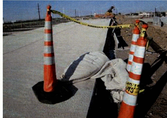
Figure 4.38 Pavement at US82 under construction
