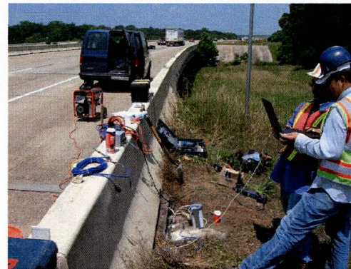
Figure 4.31 Location of crackmeter installation
