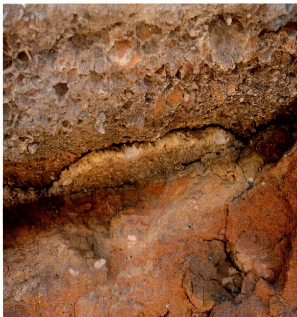
Figure 2.21 Undersealing material
