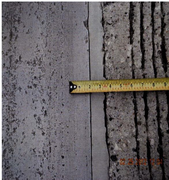
Figure 2.24 Joint width of 1.5-in in wide flange terminal
