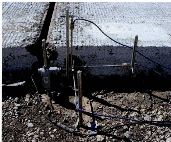
4.59 Installation of crackmeter
