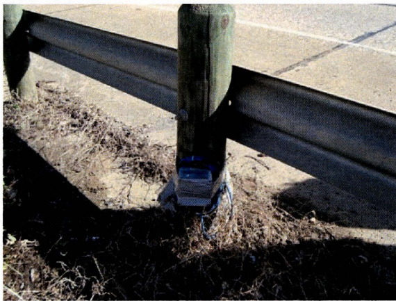
Figure 4.35 Datalogger installation
