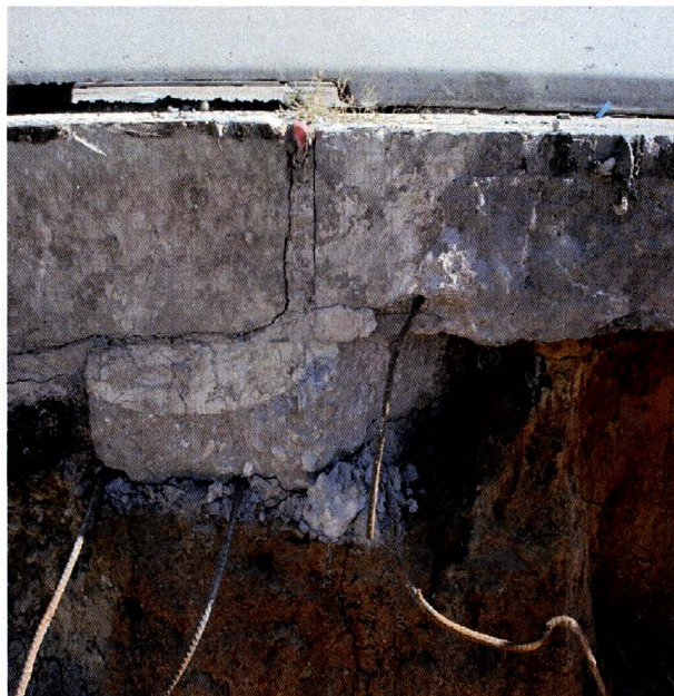
Figure 2.23 Expansion joint with support slab
