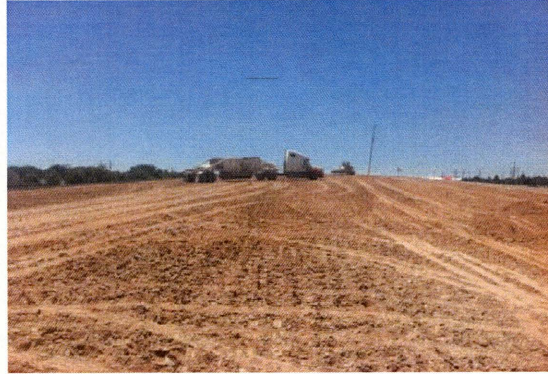
Figure 4.41 Subbase type 6 inches CSB
