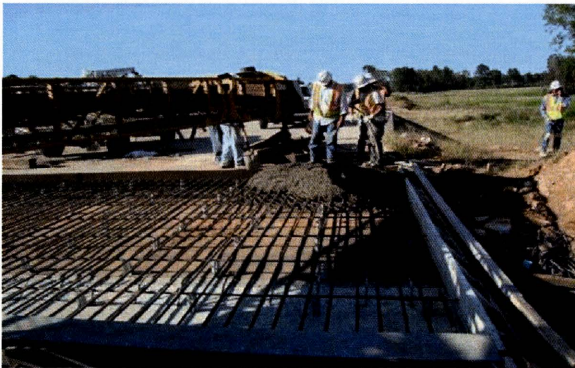
Figure 4.22 Pouring of concrete at the section
