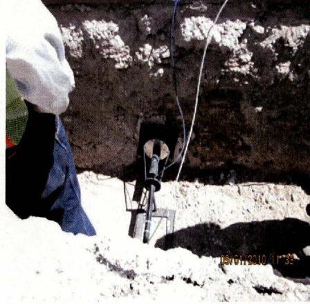
Figure 4.10 Installation of pressure cell in the AL
