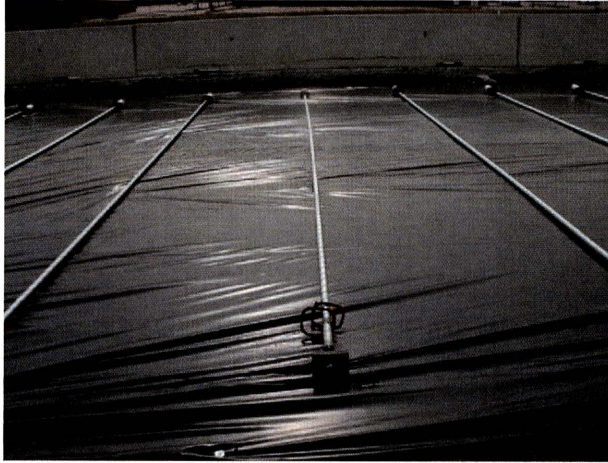
Figure 4.56 Polyethylene sheet placed between subbase and CRCP
