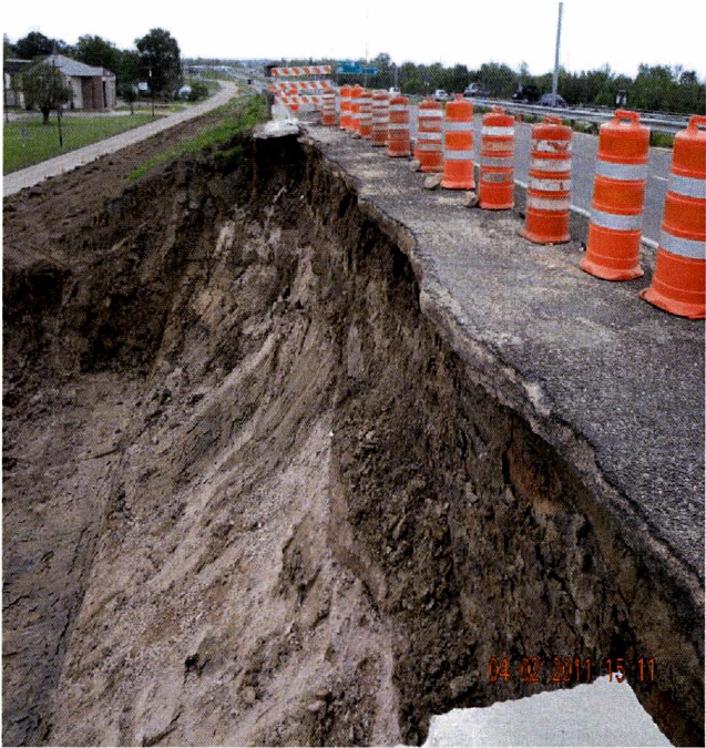
Figure 2.4 High PI clay in the embankment
