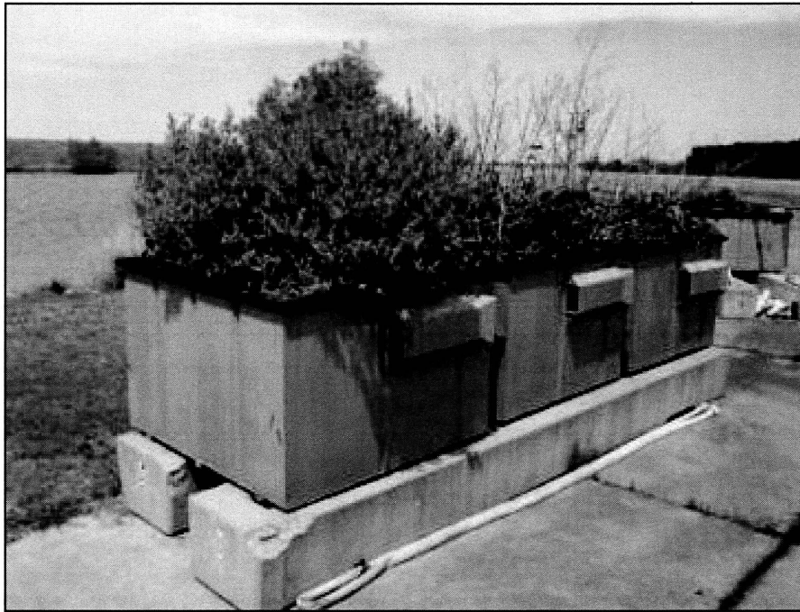
Figure 3. Bioretention Cells.
