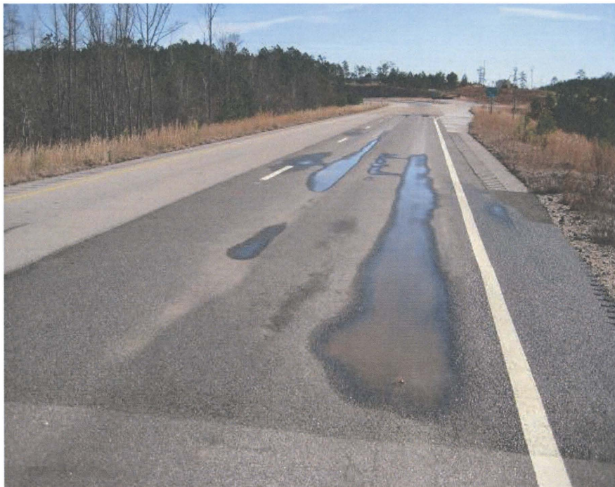
Figure 8.4: Rutting and water ponding in NCAT S12 section
