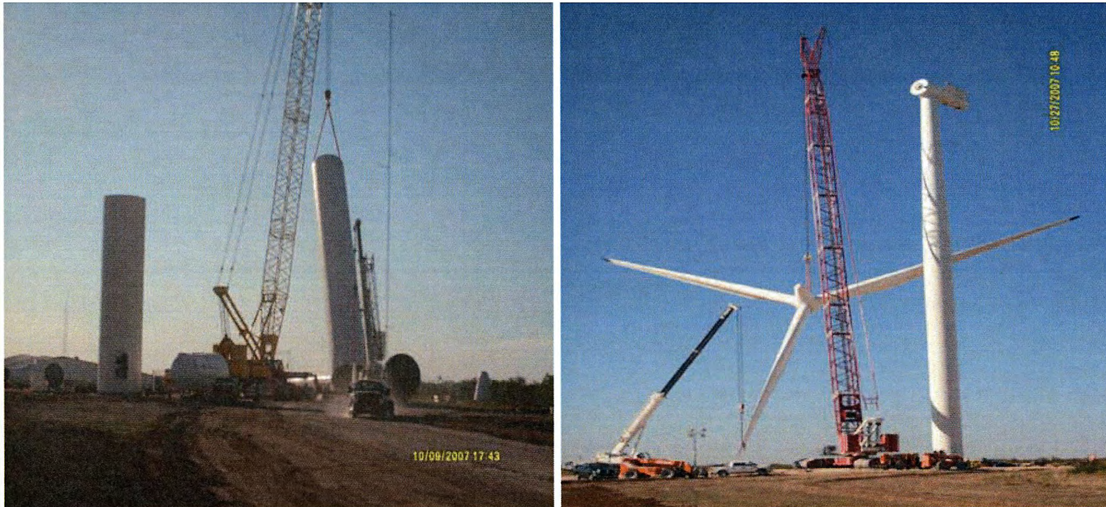
Figure 2.44: Assembly of a Wind Mill
