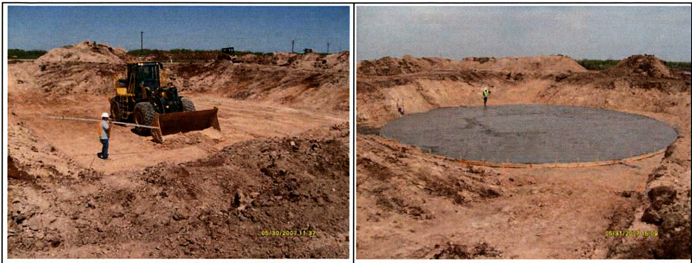
Figure 2.42: Site Preparation (Excavation and Mud Mat)
