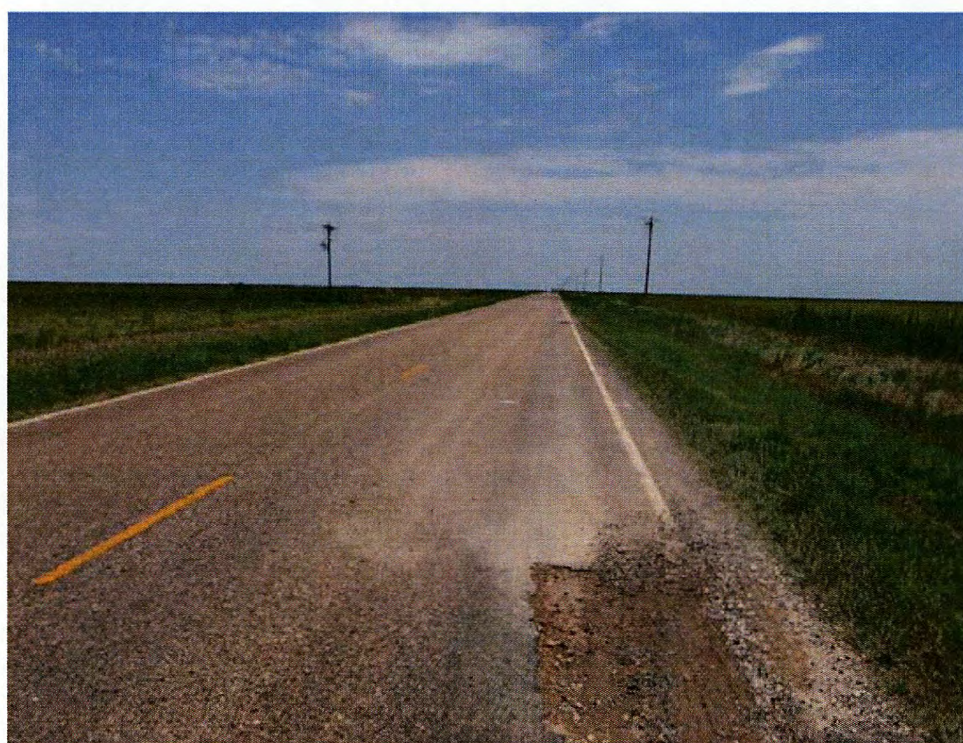
Figure 2.45: Damage on FM 97 Resulting from Windfarm Development
