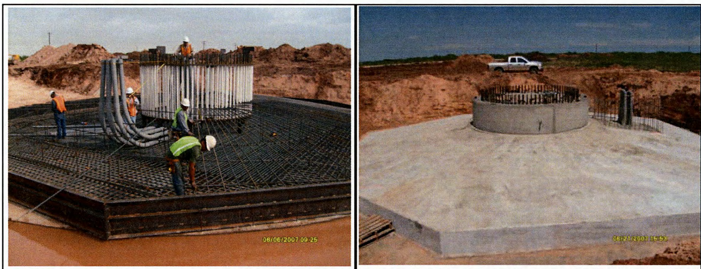
Figure 2.43: Foundation Construction Process
