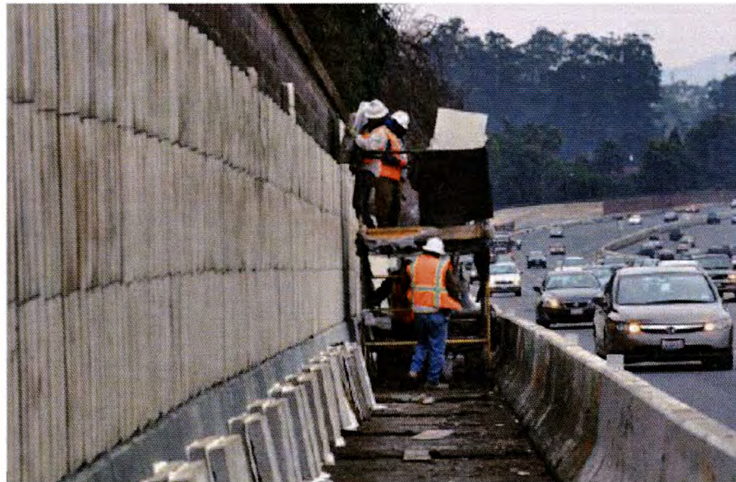
Figure 2.3: Caltrans retrofit project on US 101 (Menge & Barrett, 2010)
