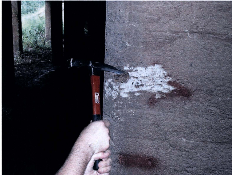
Figure 4. Hammer Test of Concrete Condition.
