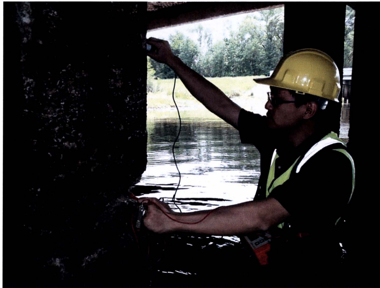
Figure 8. Half-Cell Corrosion Potential Test.
