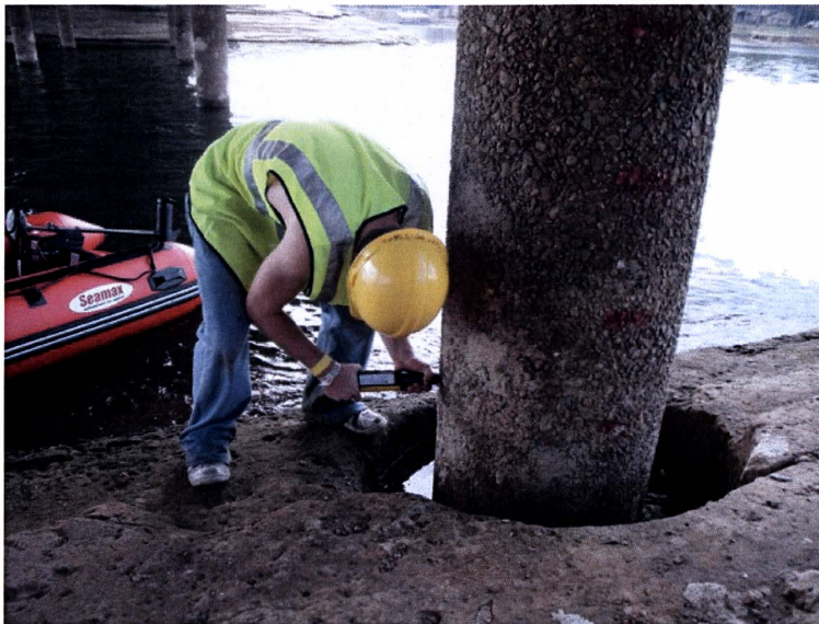
Figure 5. Schmidt Rebound Hammer Test.
