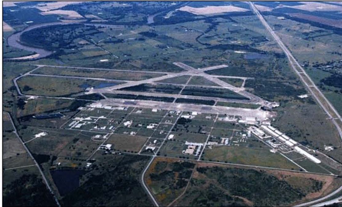
Figure 4. Riverside Campus Test Facility.
