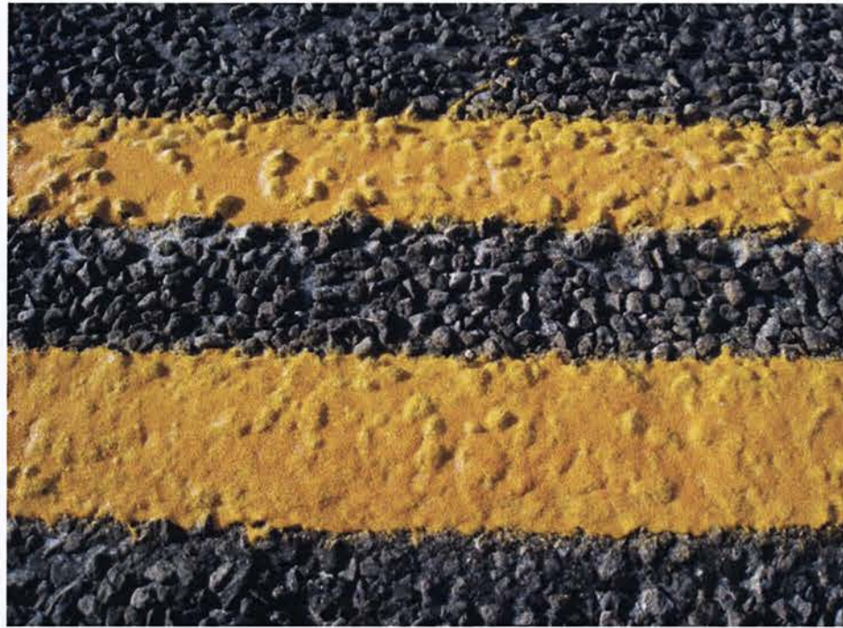
Figure 11. SH 85 Road Surface with Marking.
