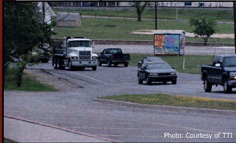
Driveway located only 150 feet from sharp Horizontal curve – inadequate sight distance.
