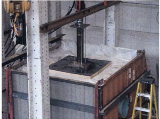
Step 10. Set up loading frame and plate.
