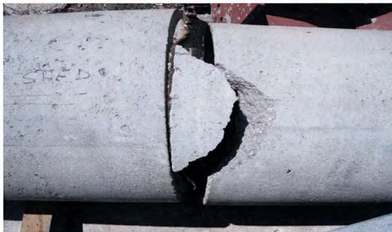
Figure 57. Concrete Pipe Fatigue Damage Observed.
