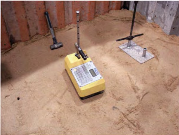
Step 3. Measure density and moisture content.
