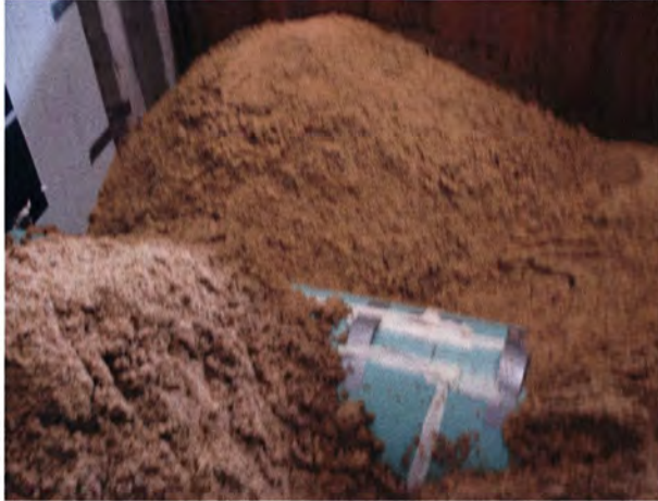
Step 7. Backfilling with sand.
