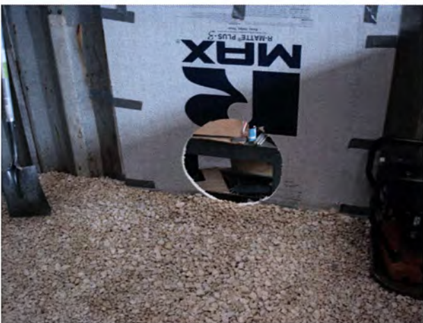
Step 5. Deposit gravel bedding layer.
