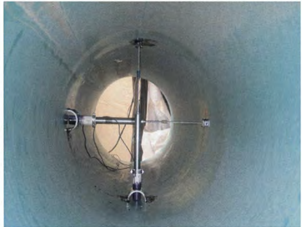
Step 12. Measure pipe deformation.
