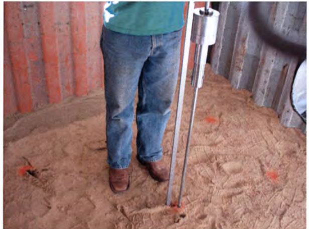
Step 4. Measure soil modulus using DCP.
