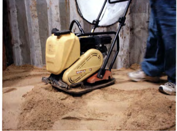
Step 2. Compact sand lift.
