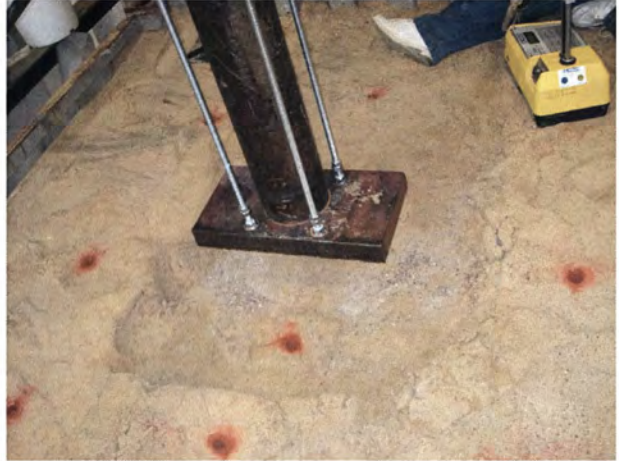
Step 8. Measure backfill density and moisture content.
