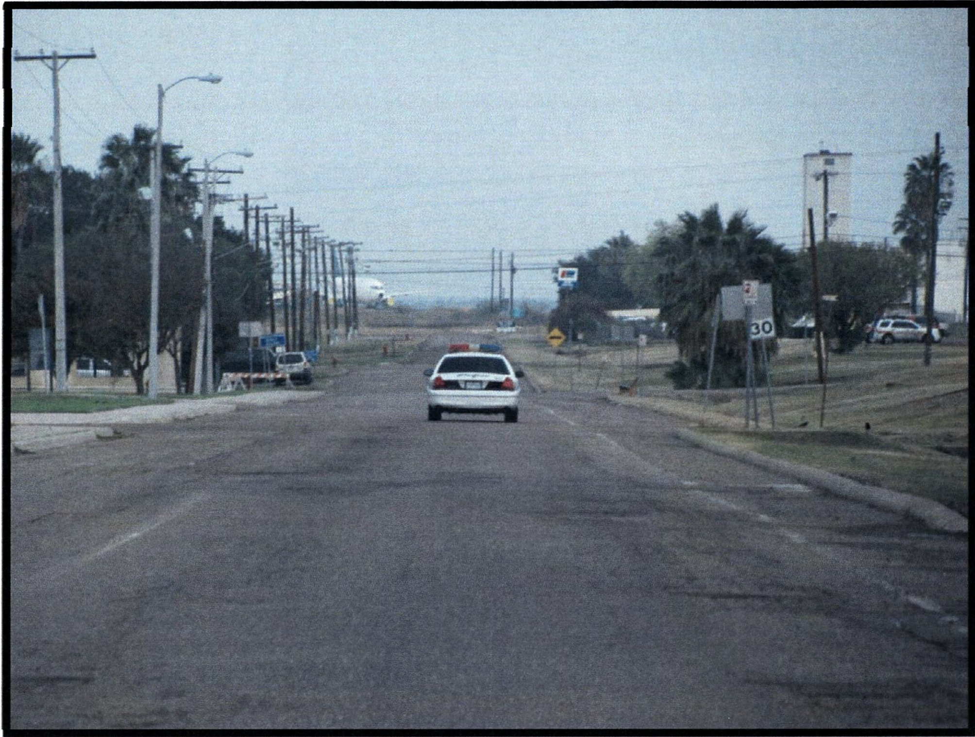
Figure 112. Laredo International Airport—Maher Avenue.
