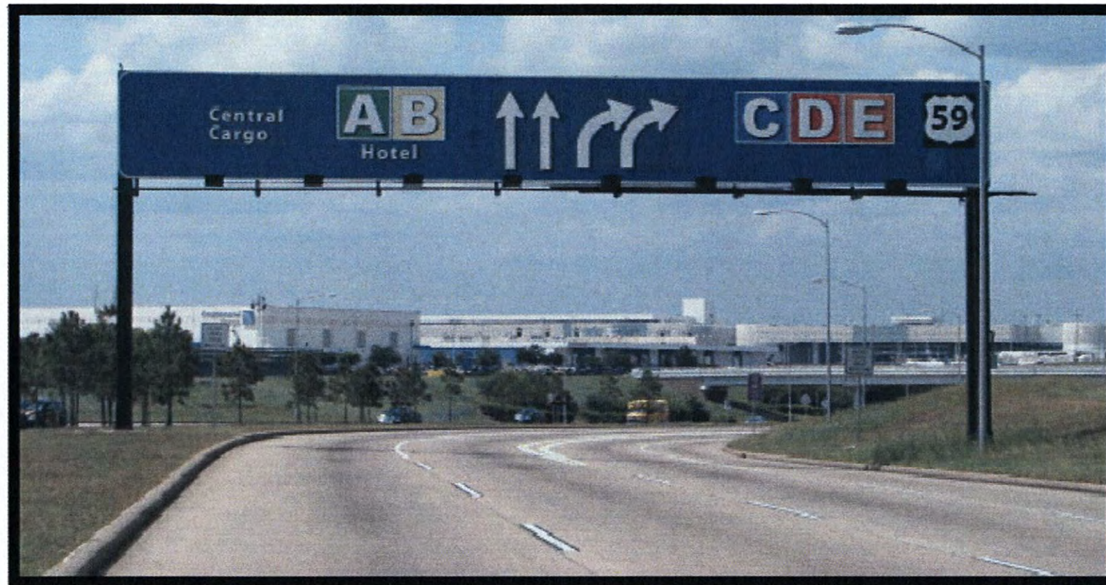
Figure 148. Freight-Area Directional Signage at George Bush Intercontinental Airport in Houston.
