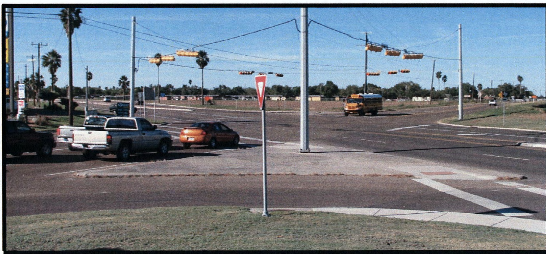
Figure 133. Skewed Intersection—SL 499 at FM 507/North 25th Street.
