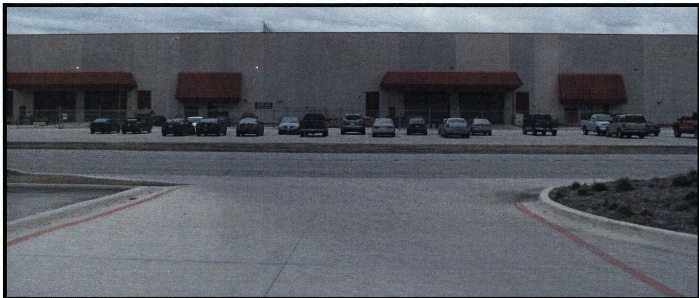
Figure 104. View of Driveway Entrance from 36th Street to the Air Cargo Facility.
