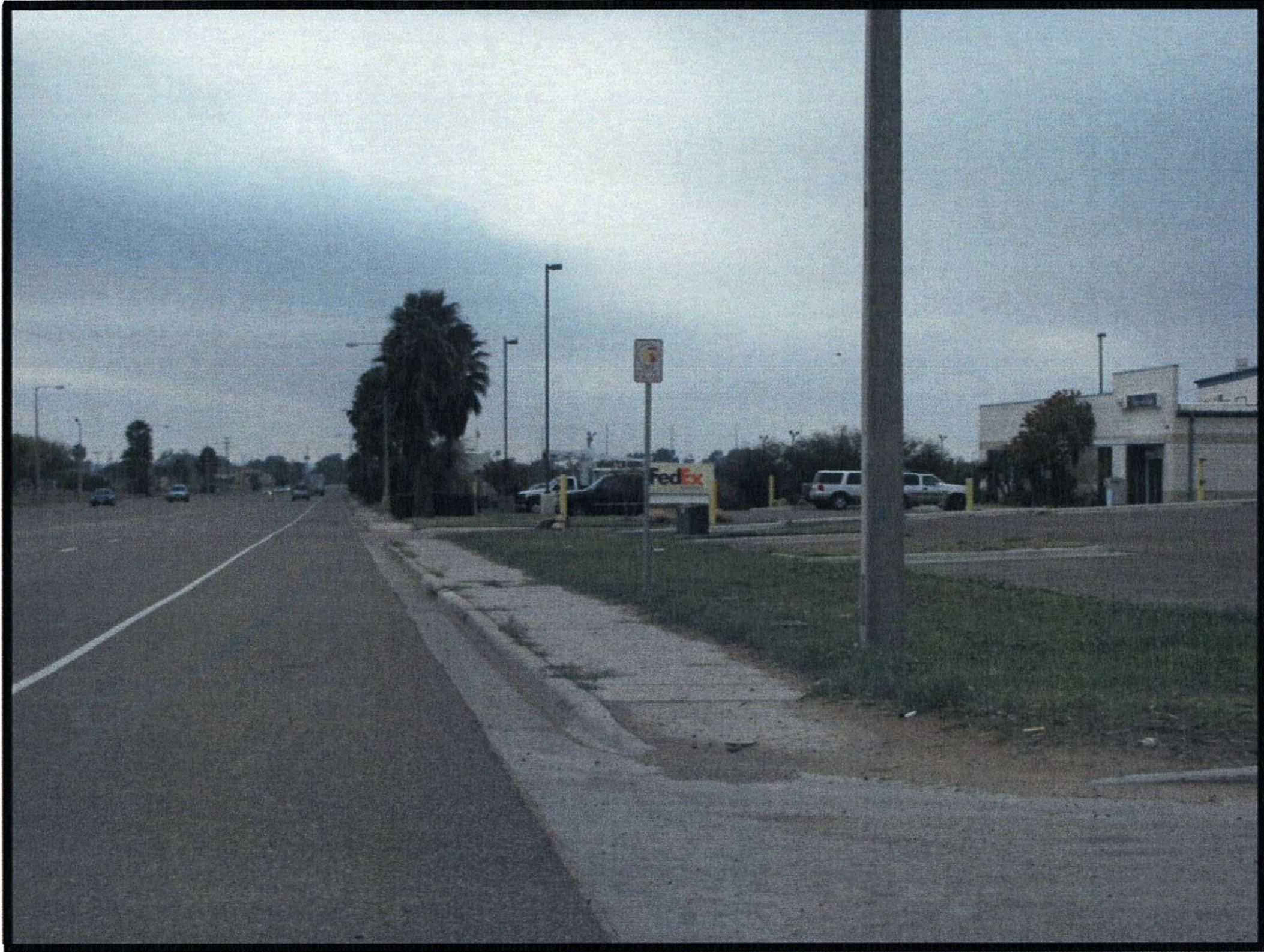
Figure 118. Laredo International Airport FedEx Cargo Facility.
