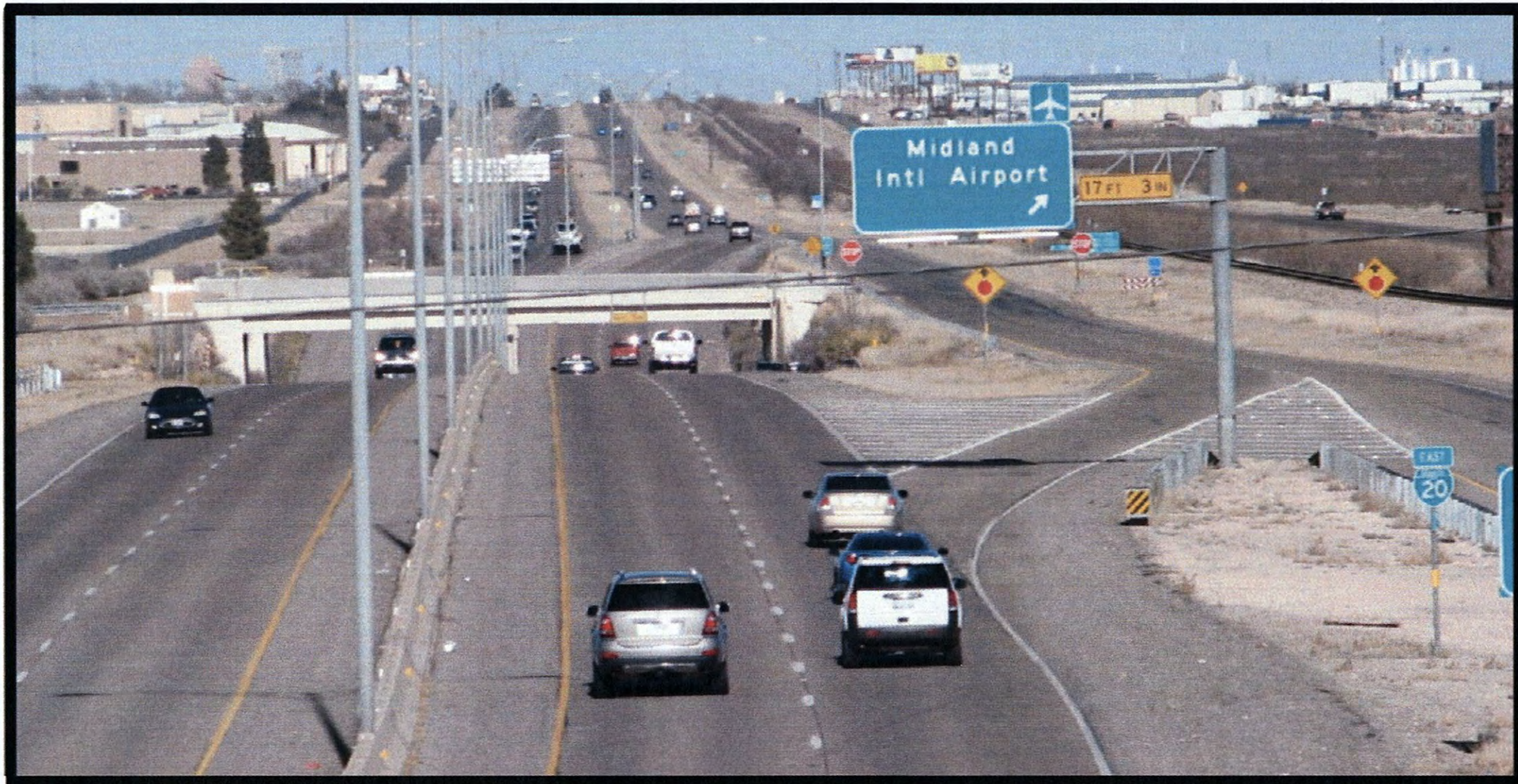
Figure 139. Exit for MAF from Eastbound BR 20.
