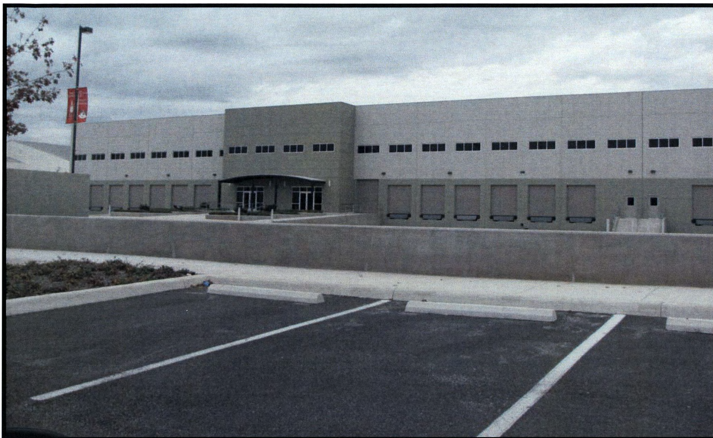
Figure 102. Landside View of the Port San Antonio Air Cargo Facility.
