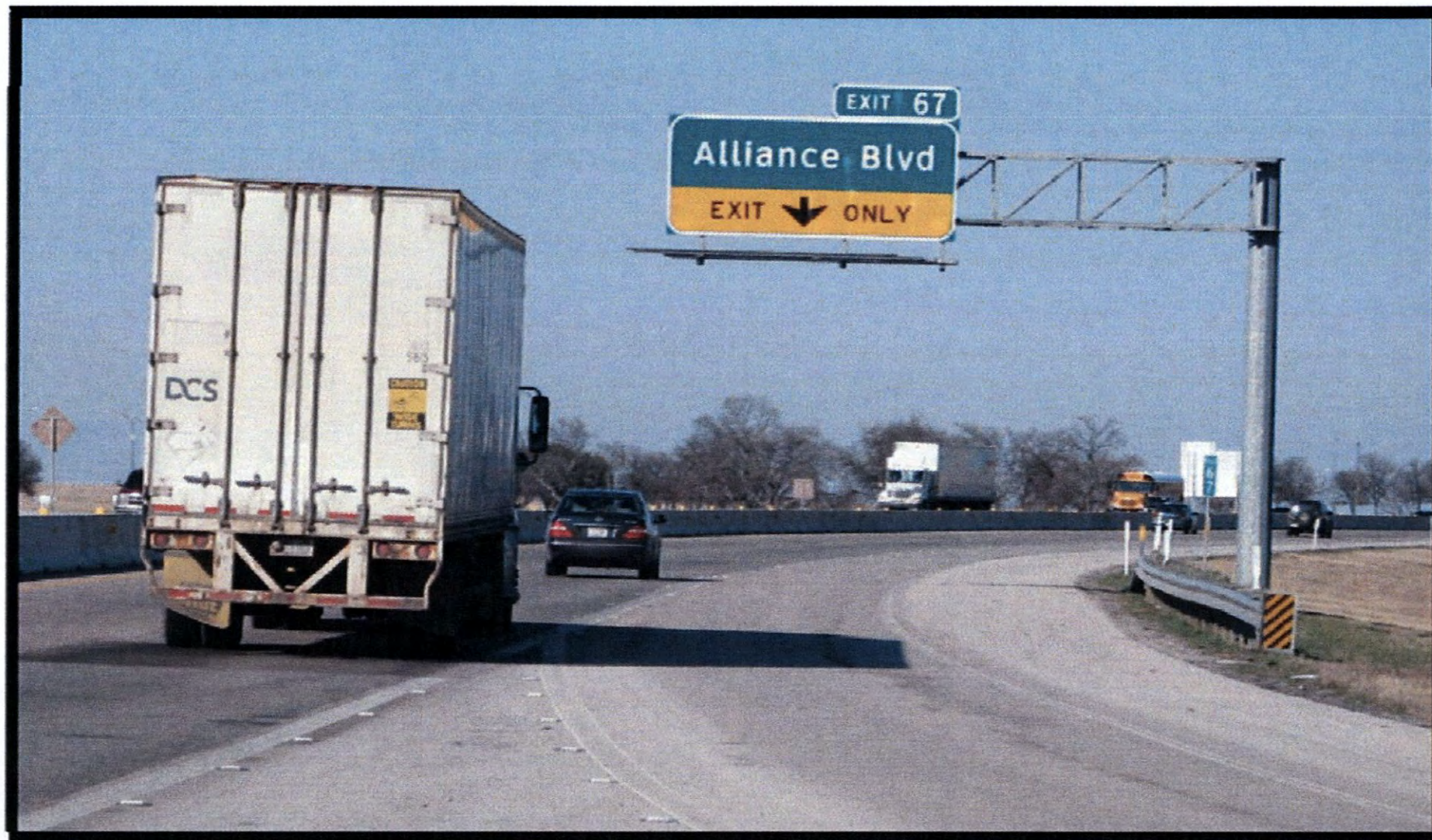
Figure 95. Exit-Only Sign for Alliance Boulevard on Northbound IH 35W.
