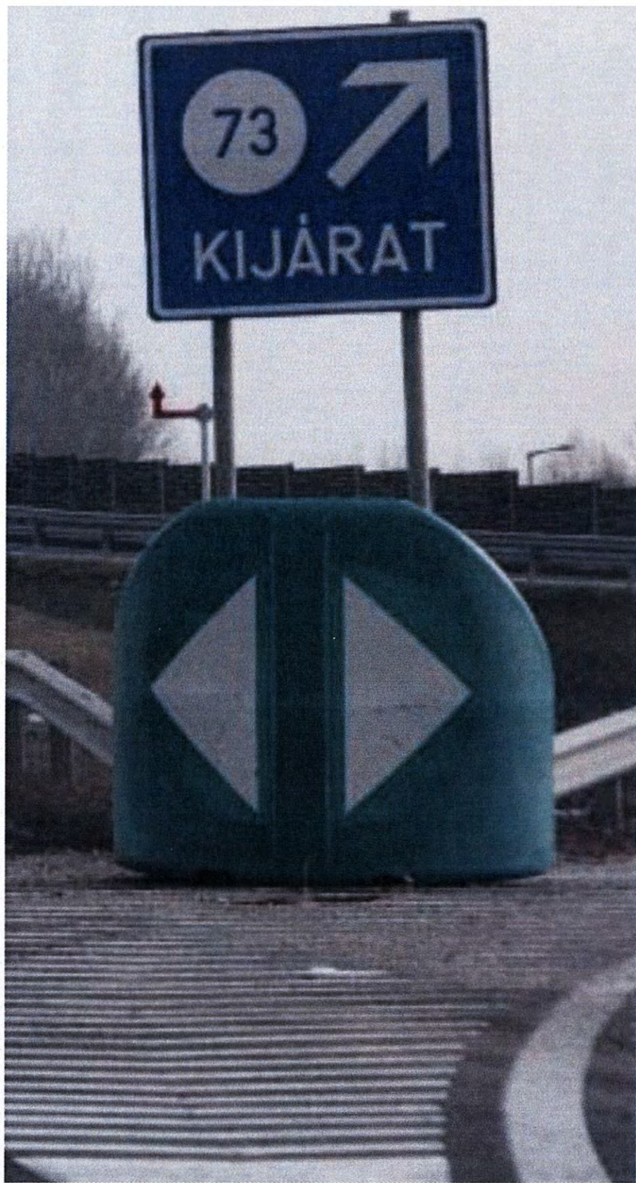
Figure 23. Impact Attenuator with Large Retro-Reflective Bi-Directional Arrows.
