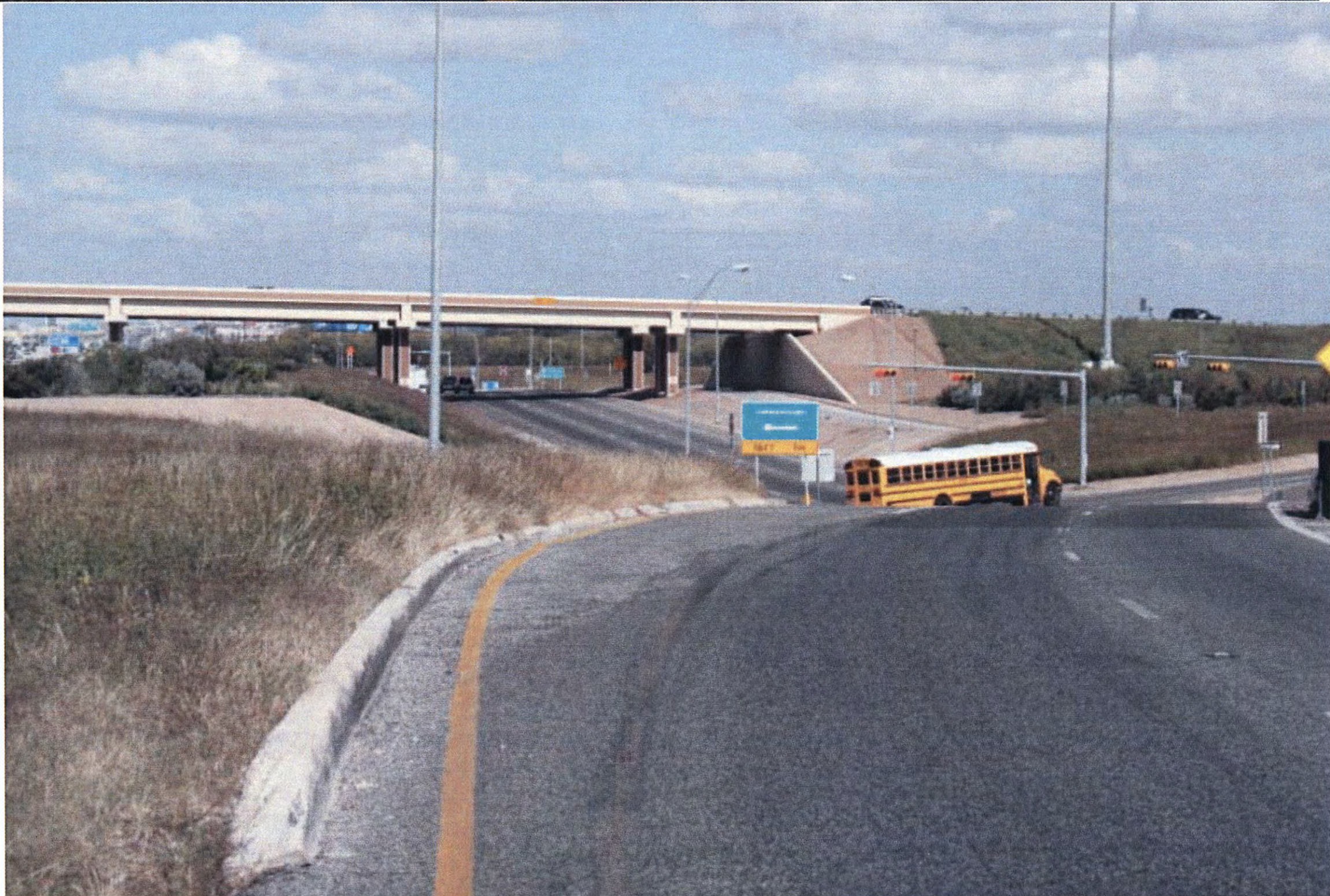
Figure 46. Northbound IH 410 Frontage Road Approach to U-Turn at SH 151.
