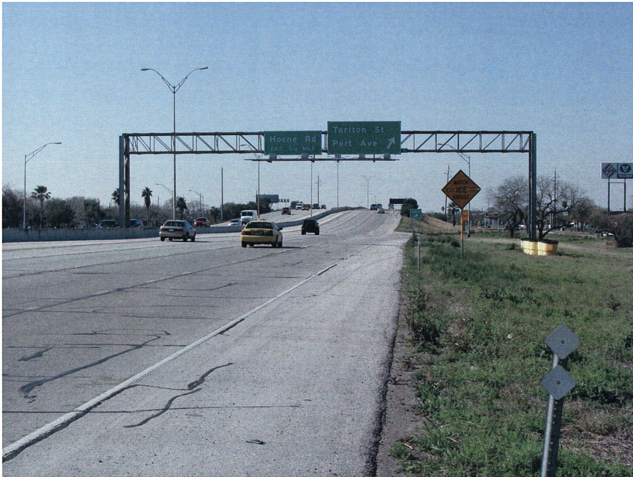
Figure 41. Southbound SH 286 Exit to Port Avenue.
