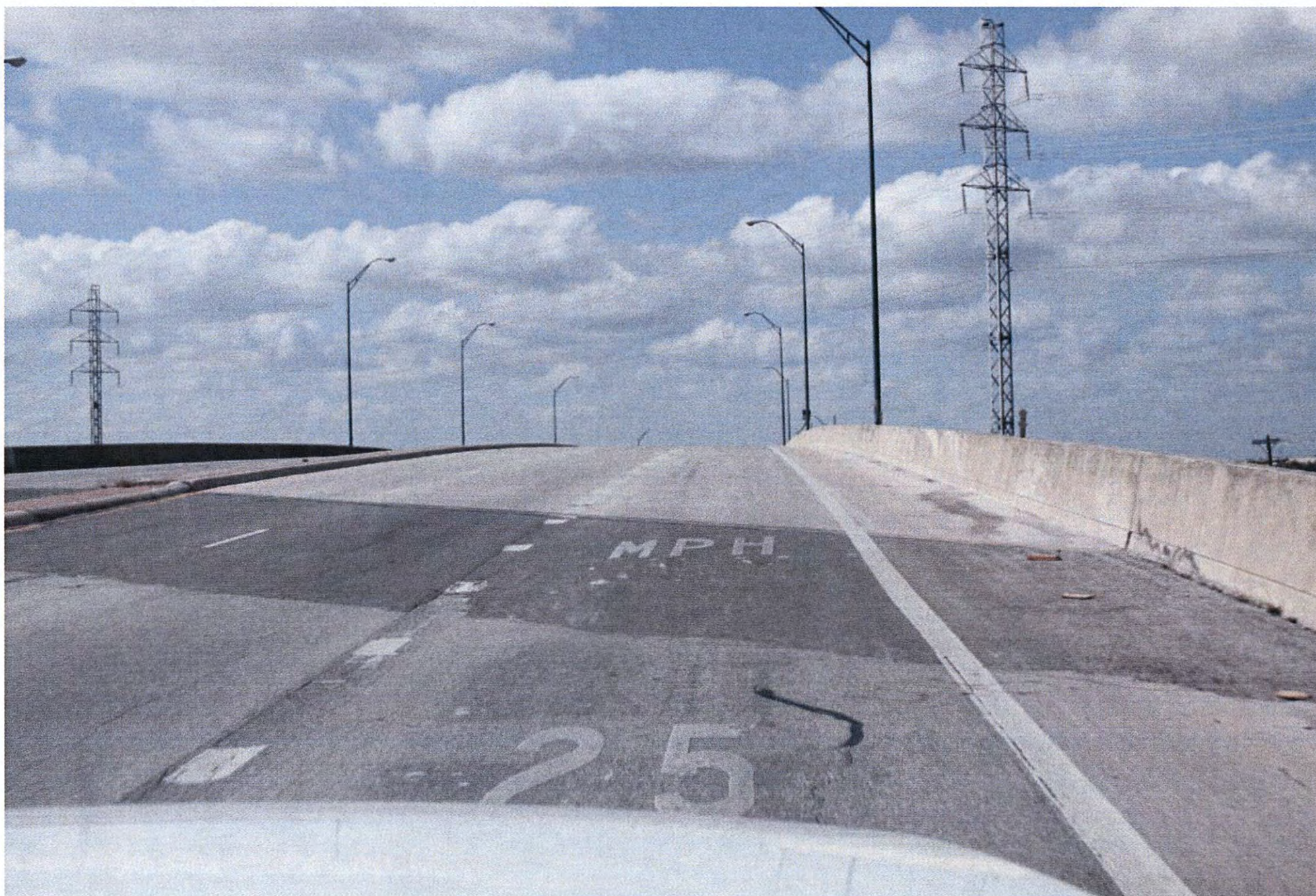
Figure 44. Example of Painted Ramp Speed on Approach to Exit on Wurzbach Parkway.
