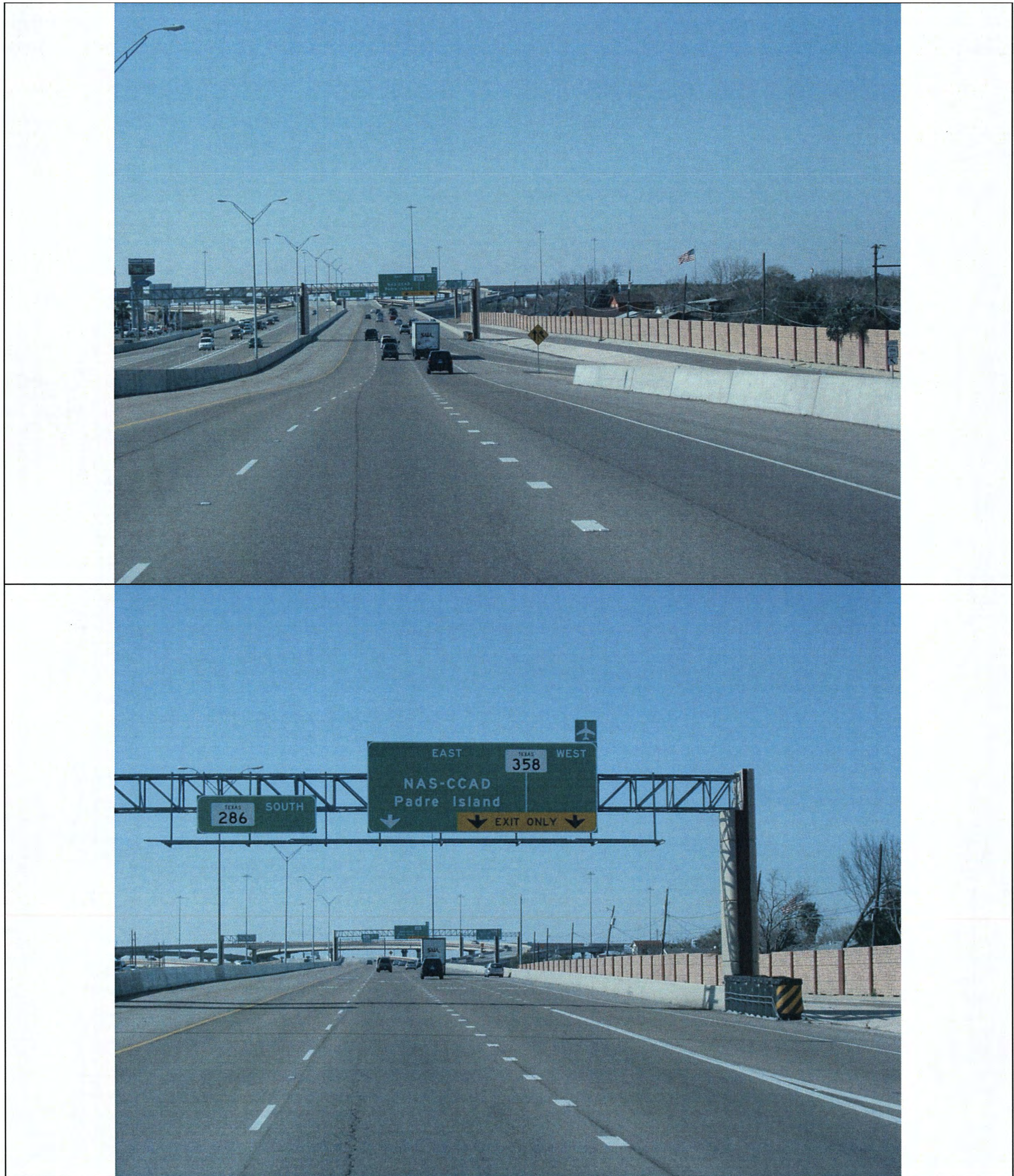
Figure 39. Approach to Southbound SH 286 Exit to SH 358 East Prior to Gore Area.
