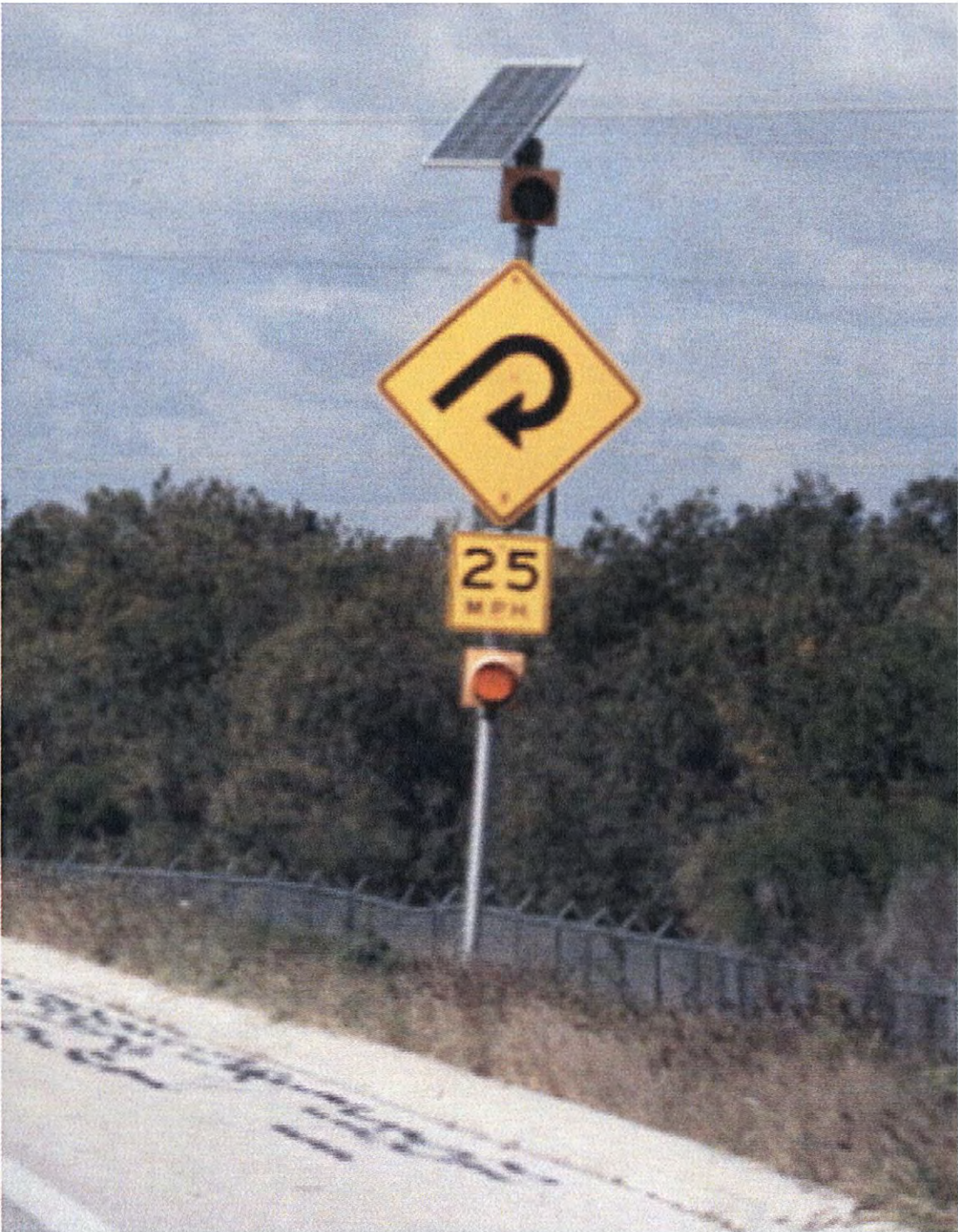
Figure 20. Advance Ramp Advisory Speed Warning Sign with Flashers.
