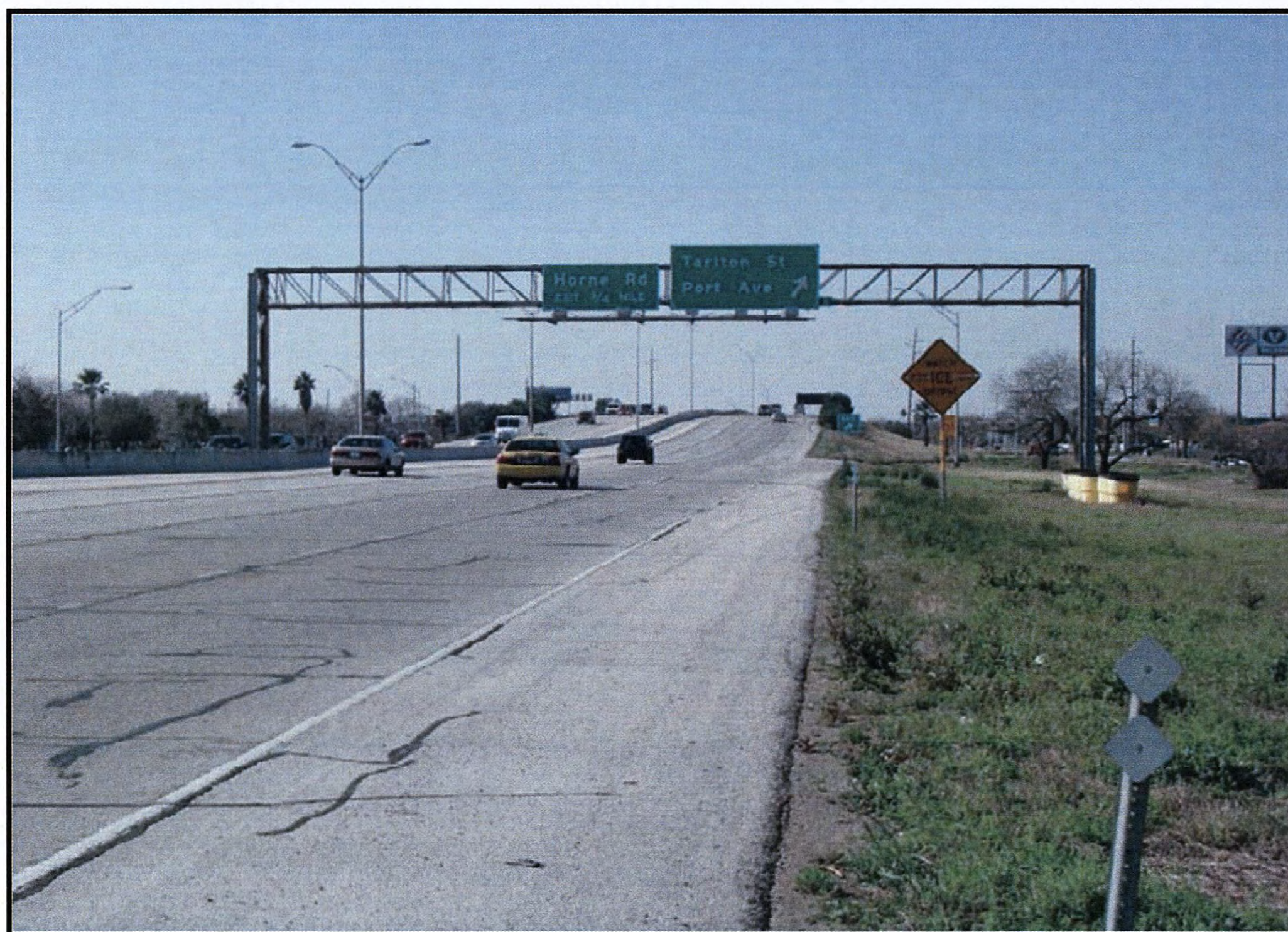
Figure 25. Southbound SH 286 Exit to Port Avenue, Corpus Christi, Texas.
