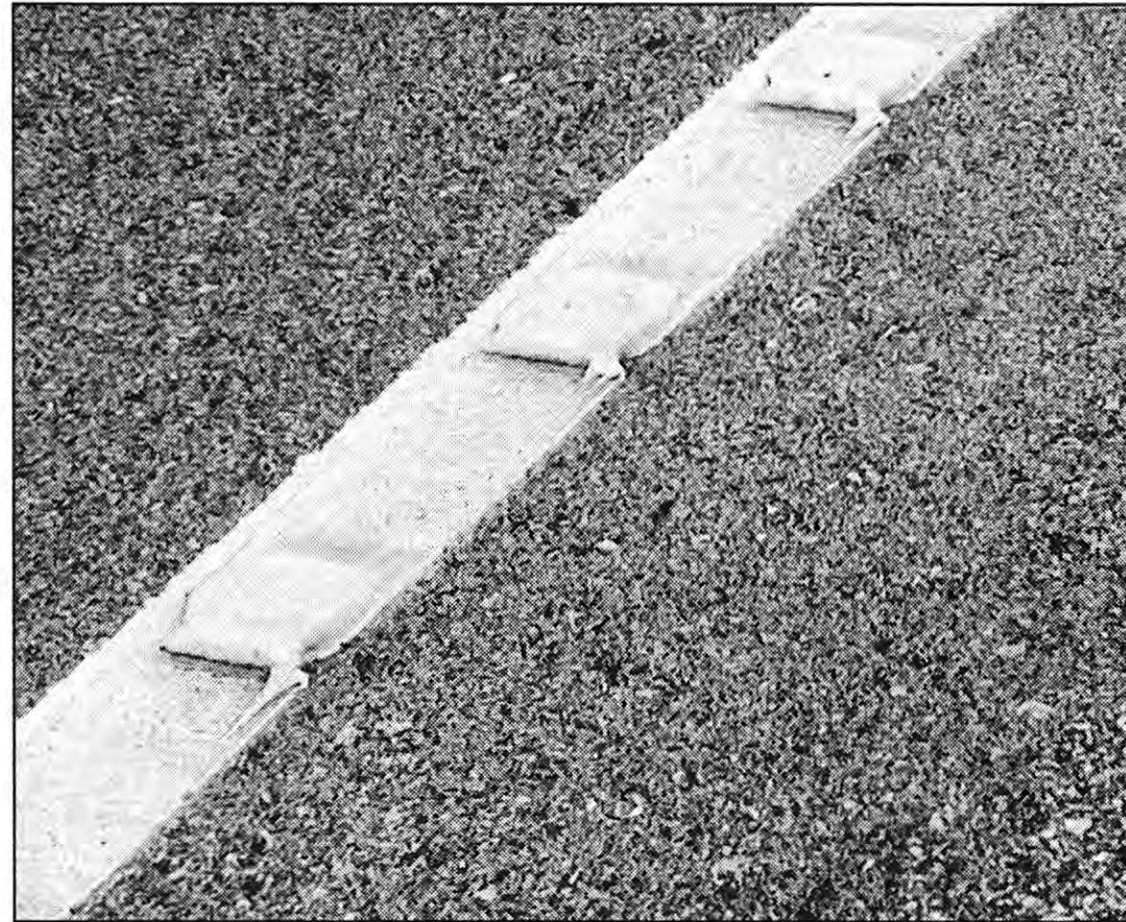
Figure 4. Profiled Pavement Marking.
