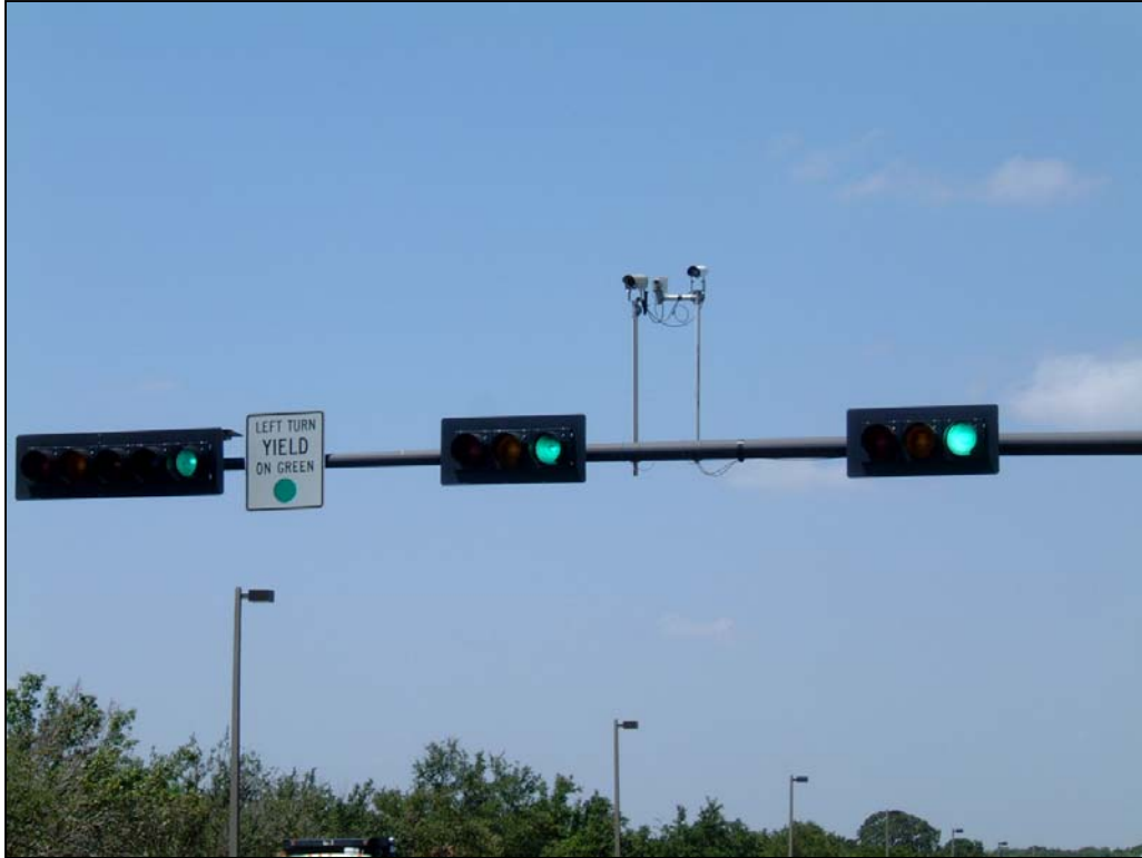
Figure 27. Mounting Arrangement of the Test Cameras.
