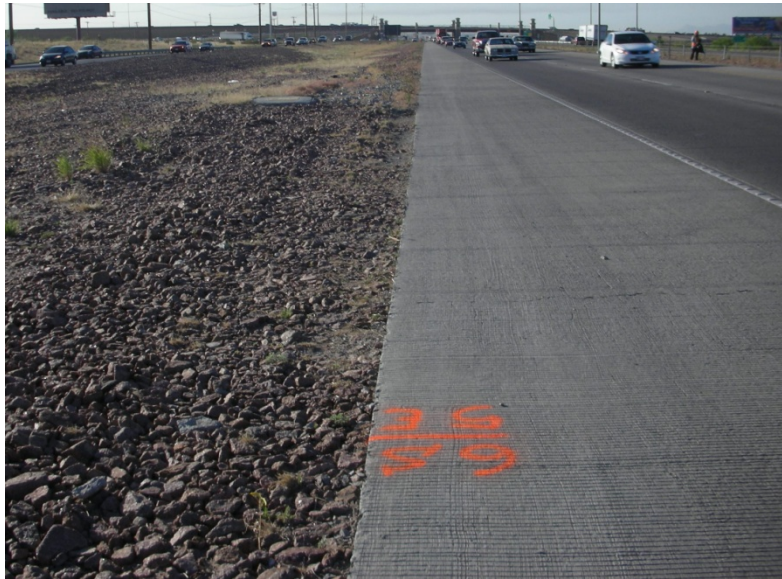
Figure 4-3. Sample Unit Limits Marked on Roadway Shoulder.
