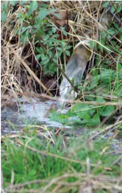
Illicit discharge in the Westfield Estates neighborhood/ photo by Justin Bower of HGAC
