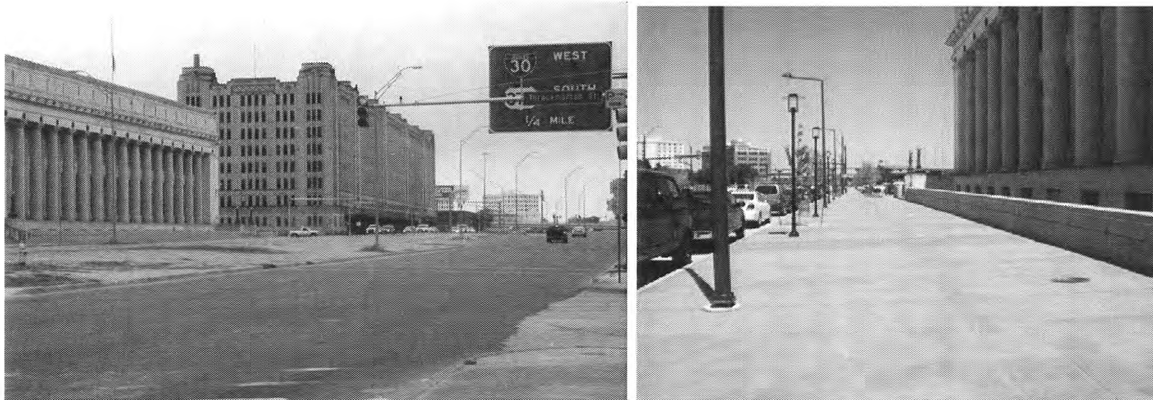
Figure 2. Before and After Photos of the U.S. Post Office Façade on Lancaster Boulevard. Source, left: http://www.durangotexas.com/eyesontexas/fortworth/downtown.htm ; Source, right: Texas Transportation Institute
