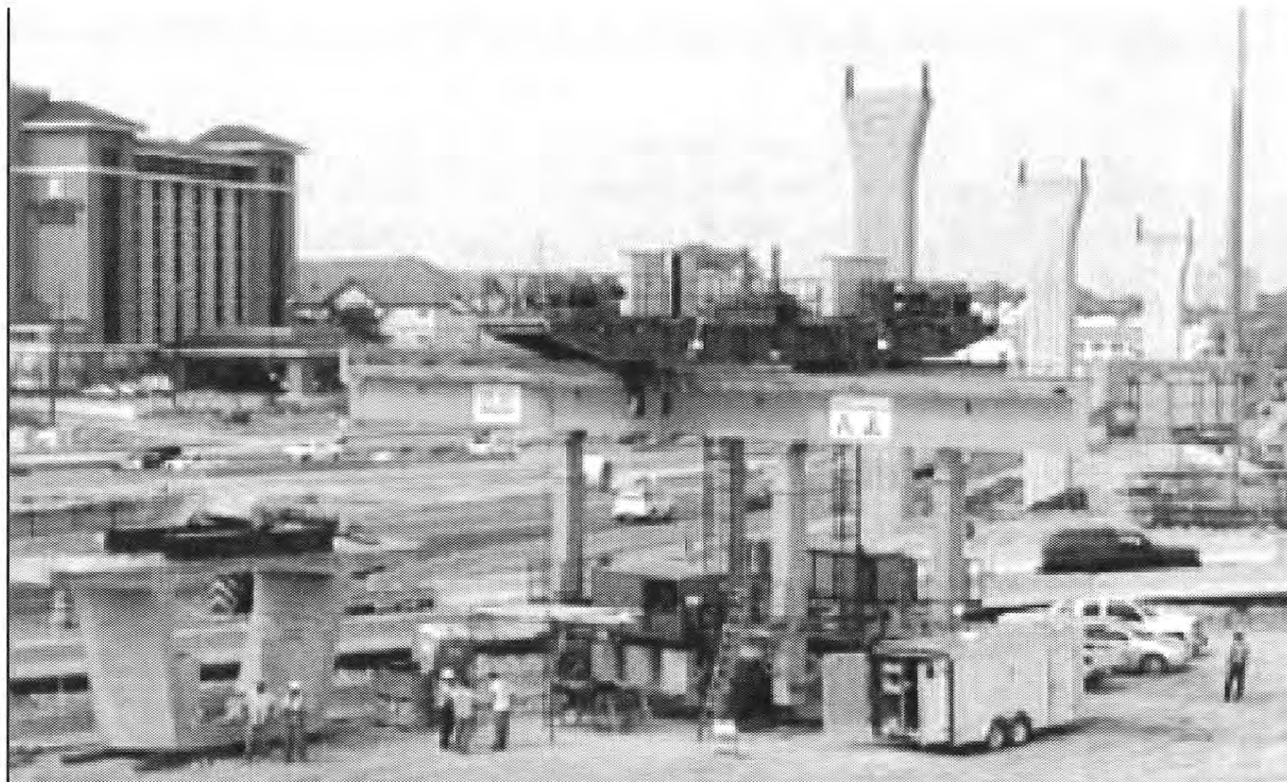
Figure 9. Segment Erector Technology.
