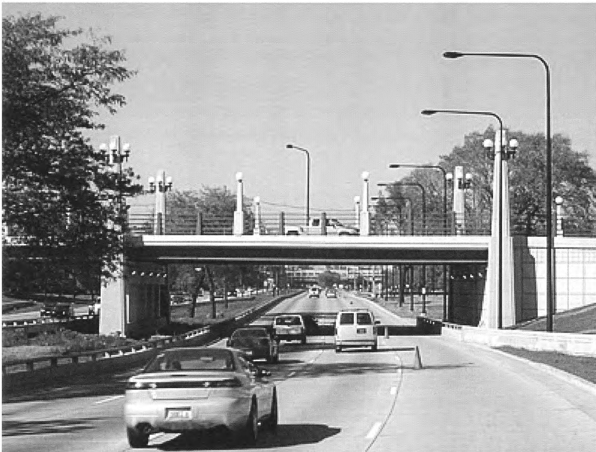
Figure 44. 31 st Street Bridge.
