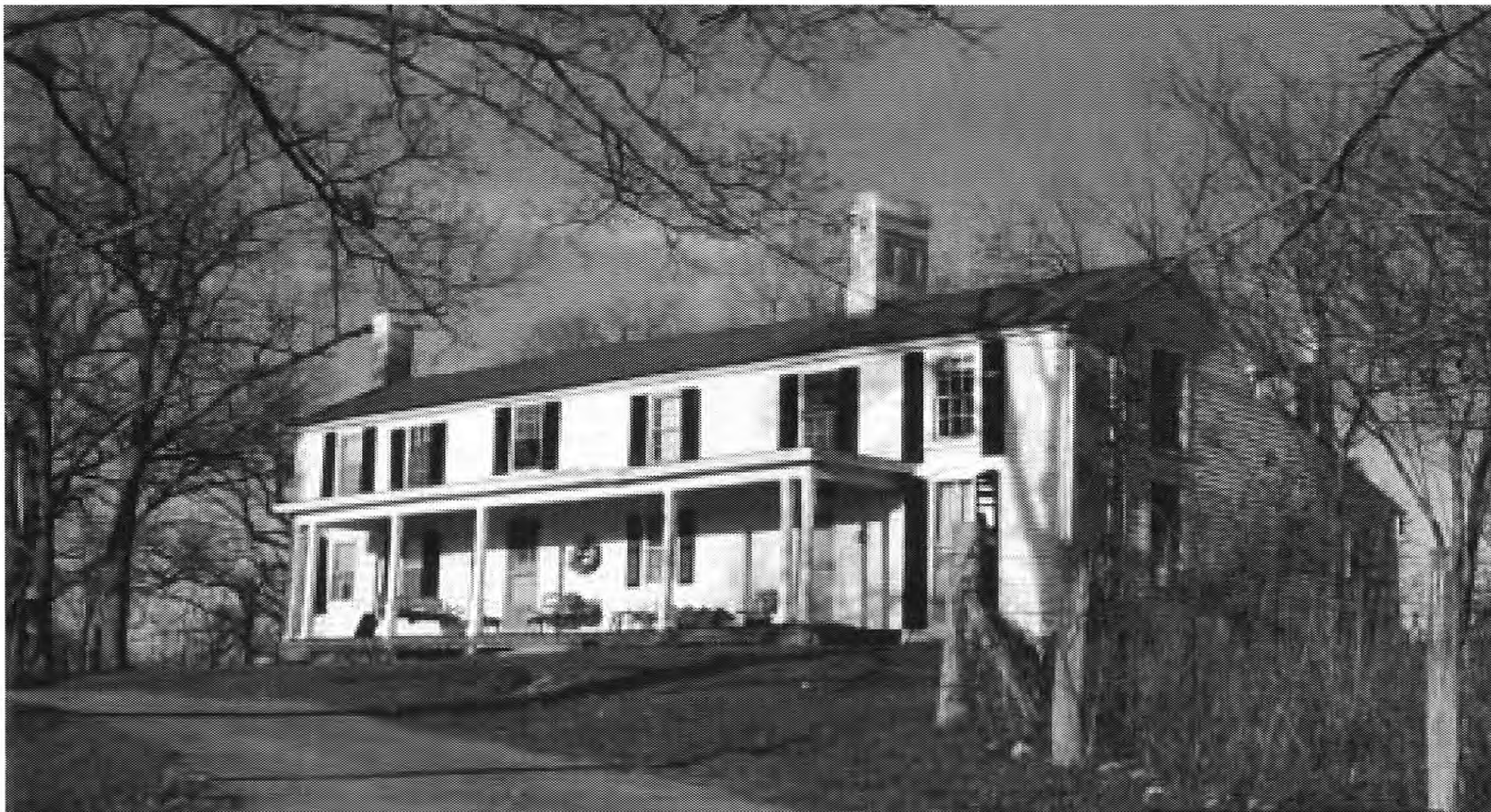
Figure 26. The Historic Wright House Was Preserved and Restored during Paris Pike Reconstruction.
