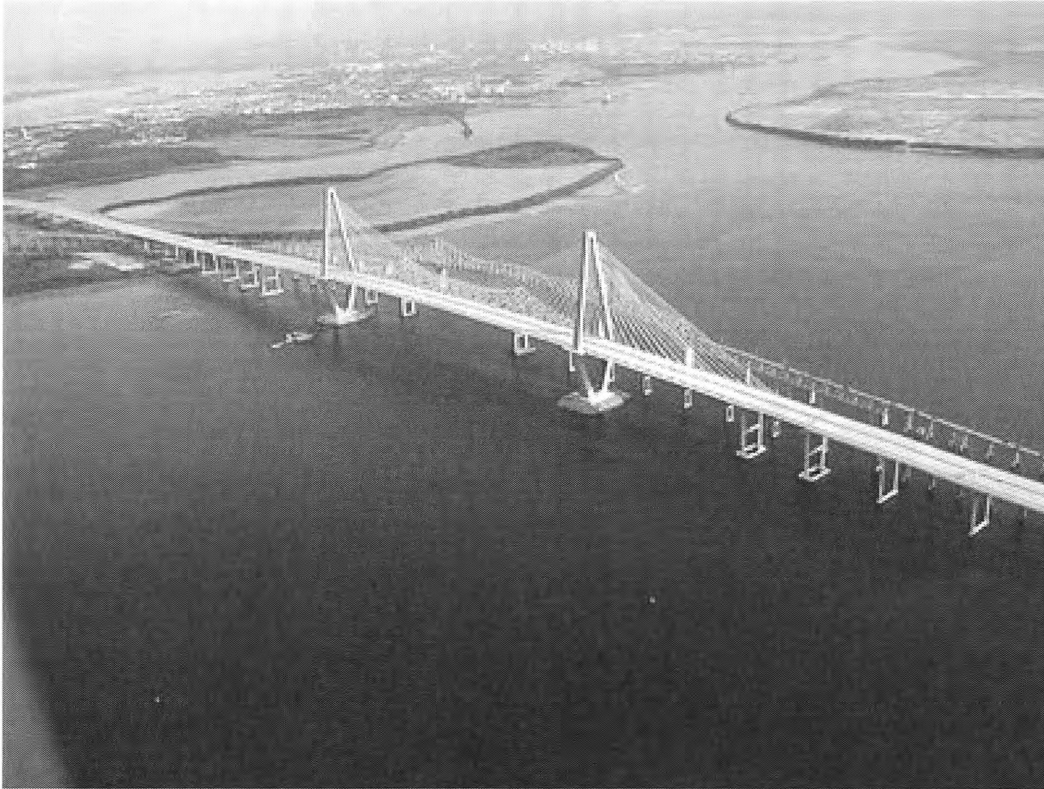
Figure 18. Cooper River Bridge Overhead Showing the Diamond Cable-Stay Design. Source: http://ravenelbridge.net/small/jul_12_bridge_south_blog.jpg
