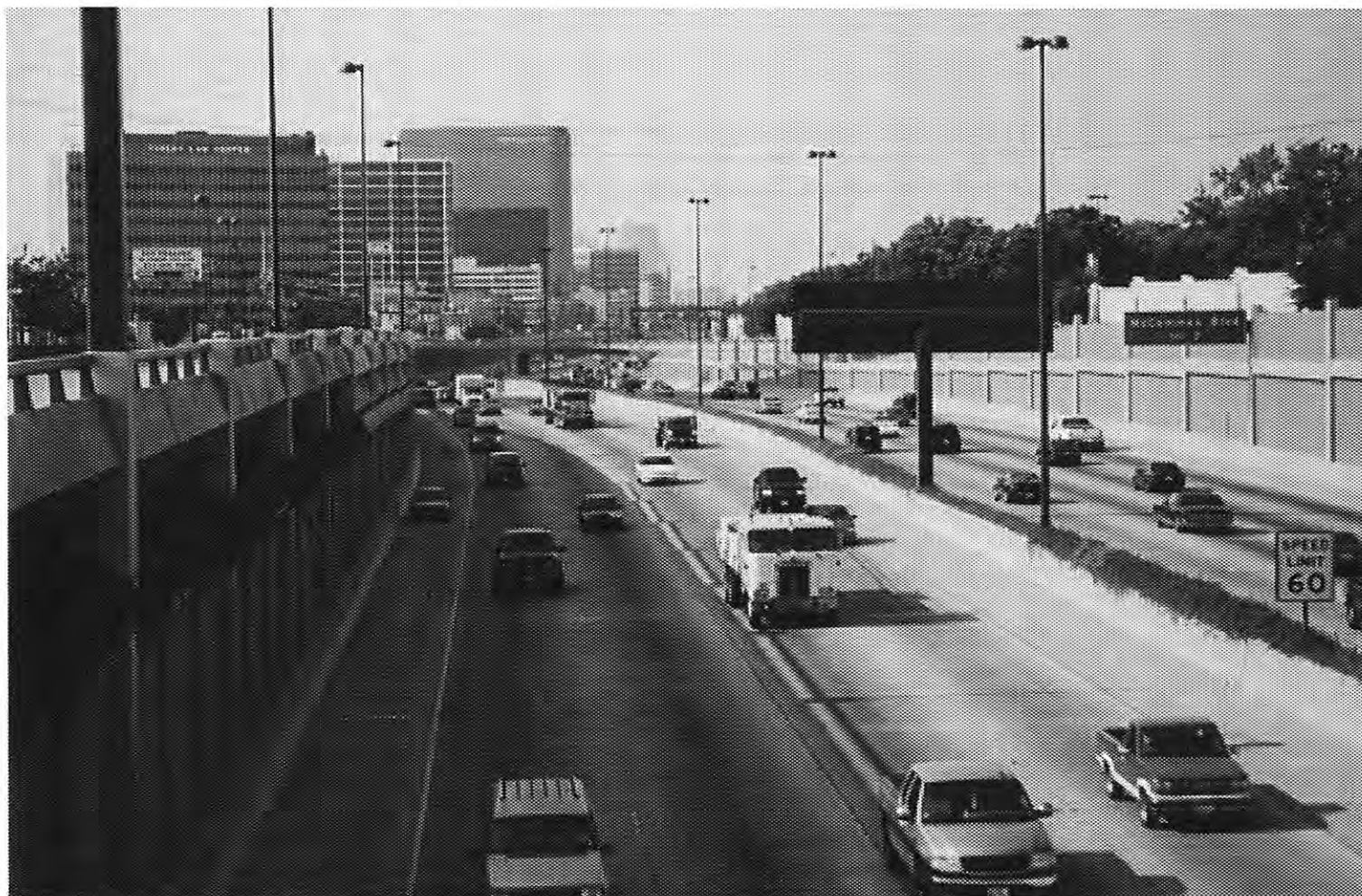
Figure 7. NC Expressway, Looking South in Depressed Section. Source: http://www.texasfreeway.com/Dallas/photos/us75/us75.shtml
