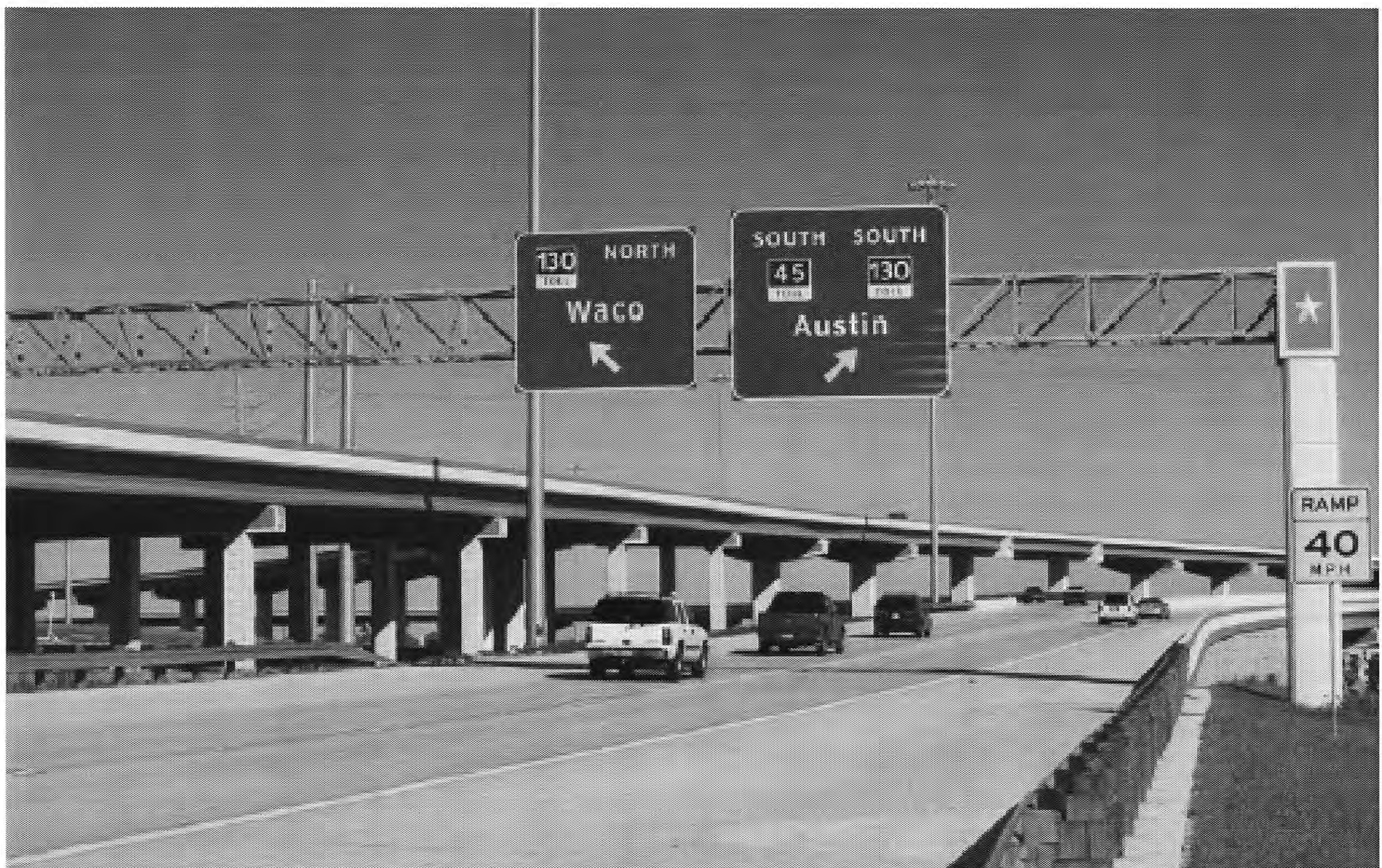
Figure 12. Appearance Features on Bridge and Sign Structures.
