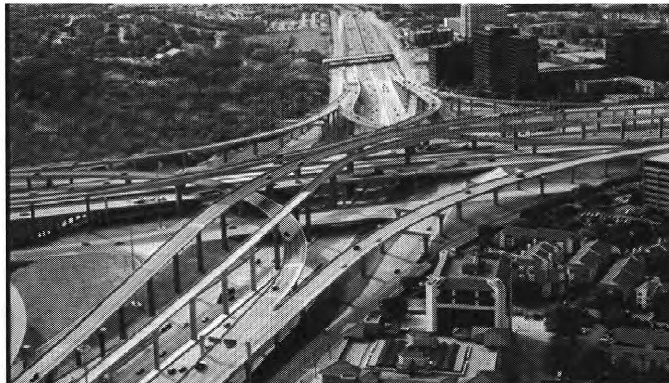
Figure 10. Completed I-635-US 75 (High Five) Interchange.
