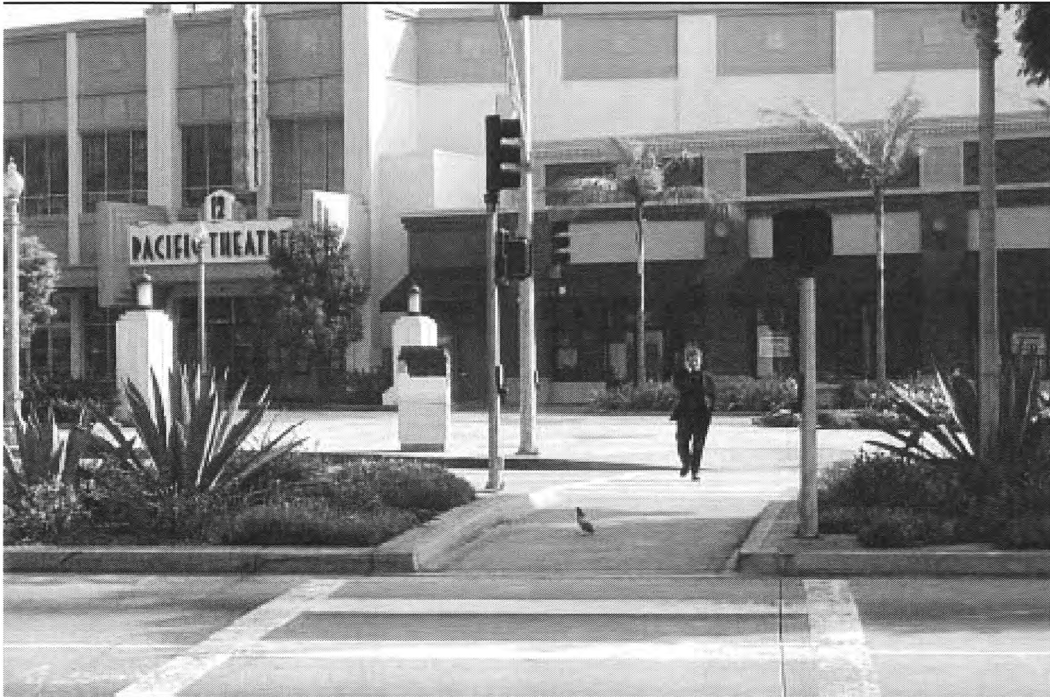
Figure 53. Culver Boulevard Streetscape and Pedestrian Friendly Crosswalks Source: Kimley-Horn and Associates, Inc.
