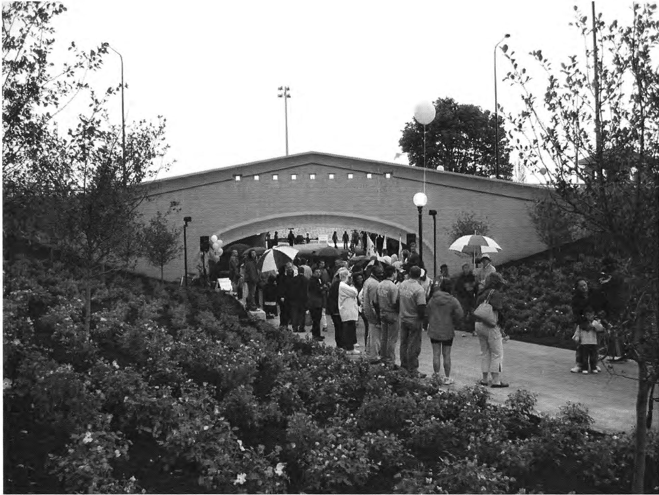
Figure 41. 63rd Street Underpass Source: City of Chicago et al.
