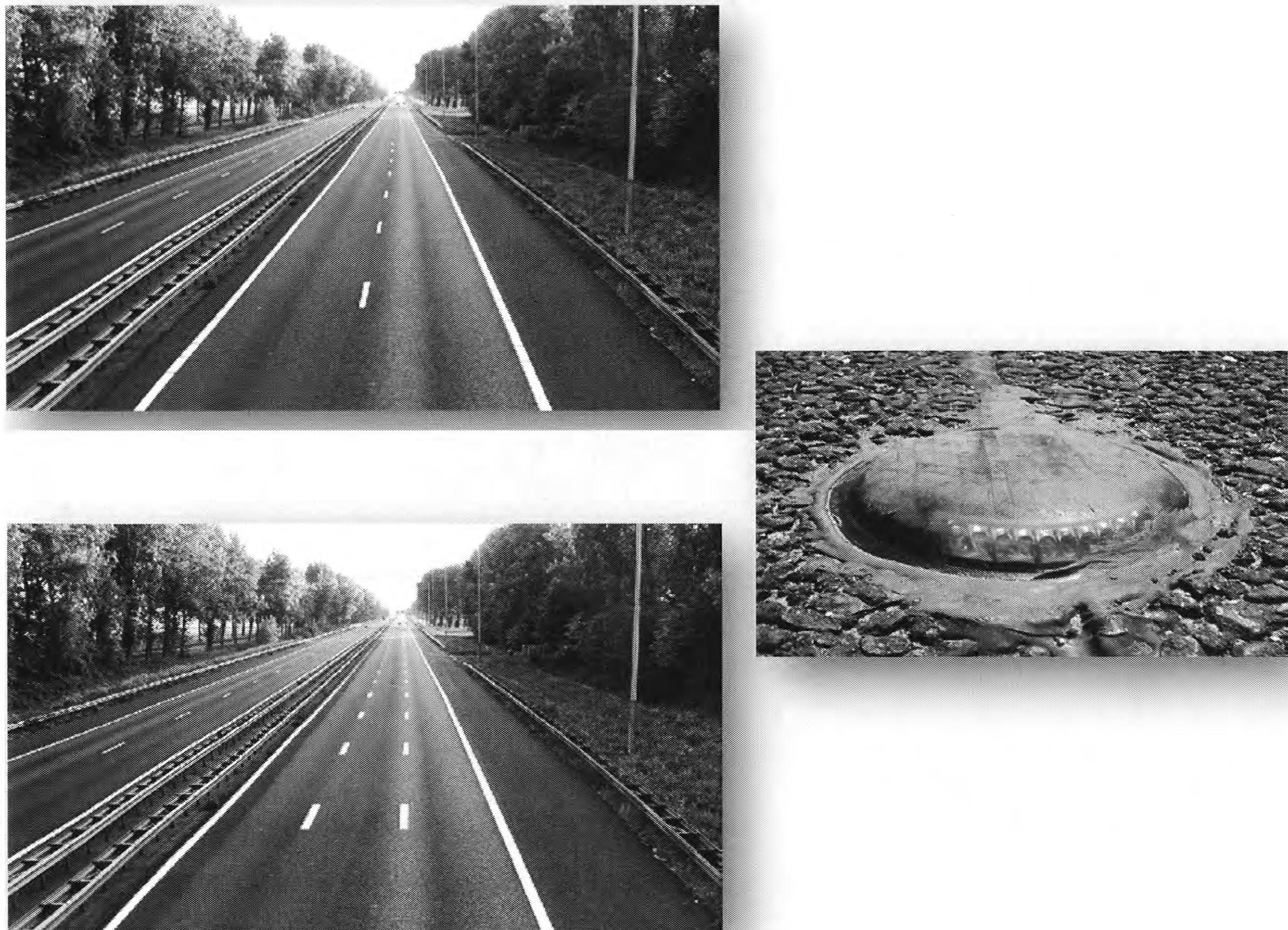
Figure 7. Left, a “flexroad” with its two possible cross sections on the A44. Right, an LED-based pavement device used for dynamic lane marking (8).
