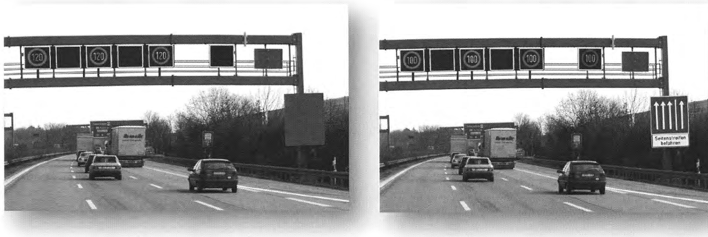
Figure 5. Hard shoulder for emergency only (left) and in use (right) (8).
