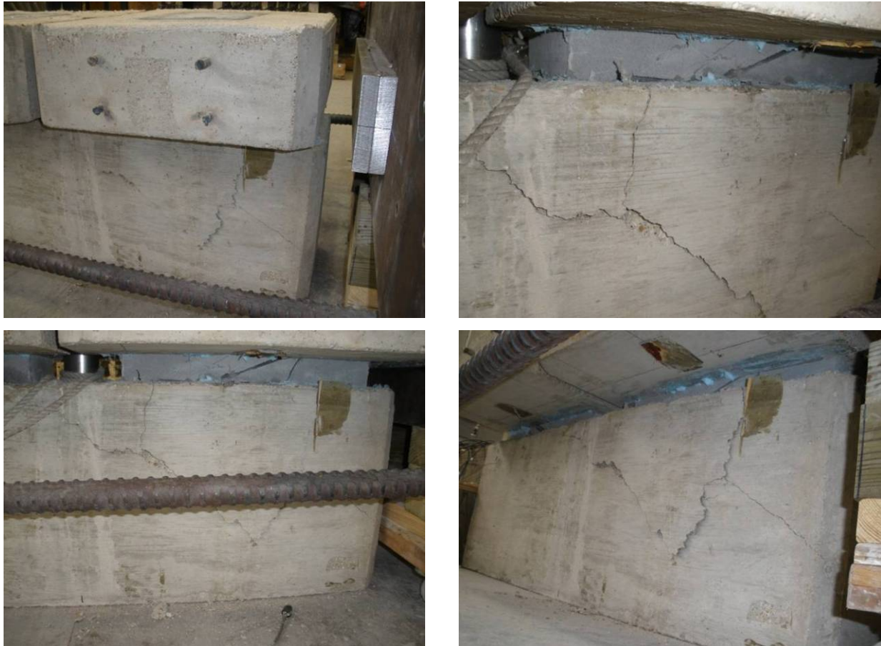
Figure 3-34. Photographs of the Cone Pullout Failure Exhibited by 2_BC_2.0.
