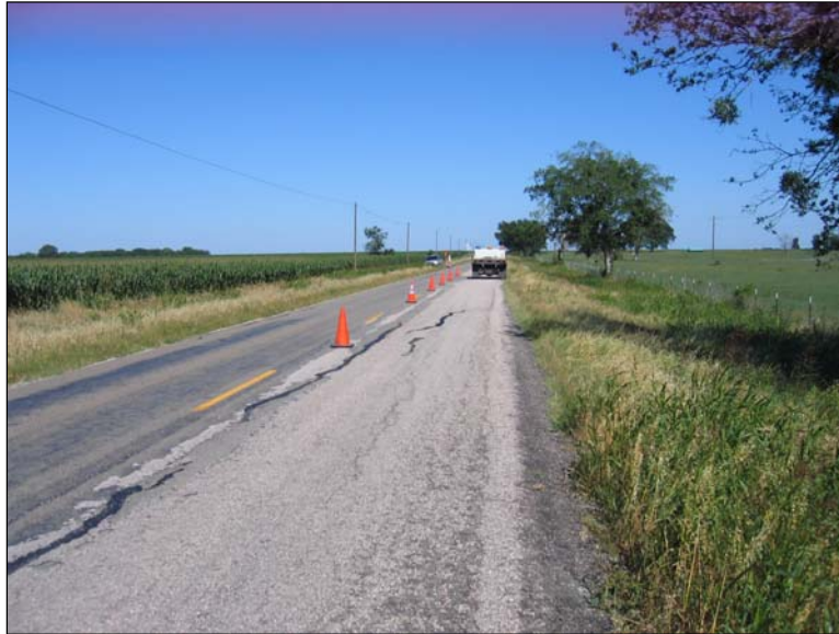
Figure 3.4. FM 487 Sampling Locations in Maintenance Location 7.
