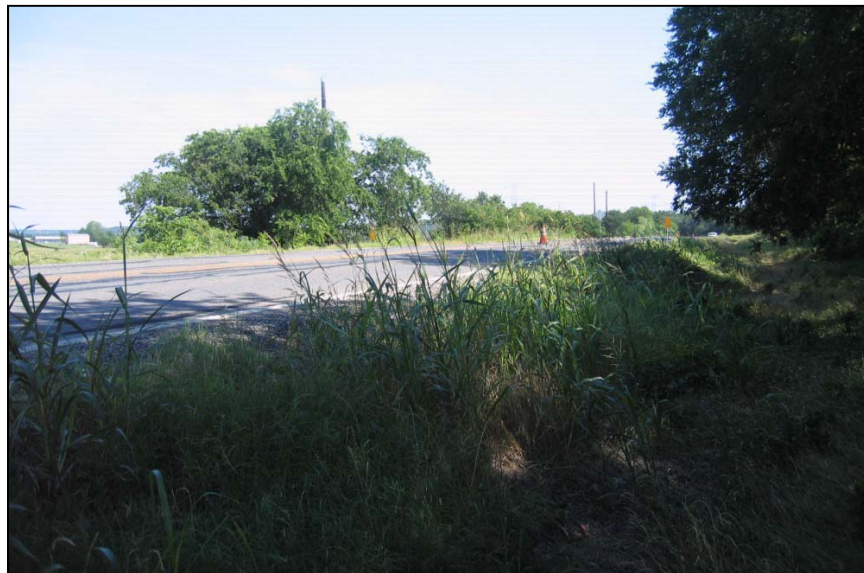
Figure 5.5. Steep Side Slopes at FM 969 Sampling Location 1.
