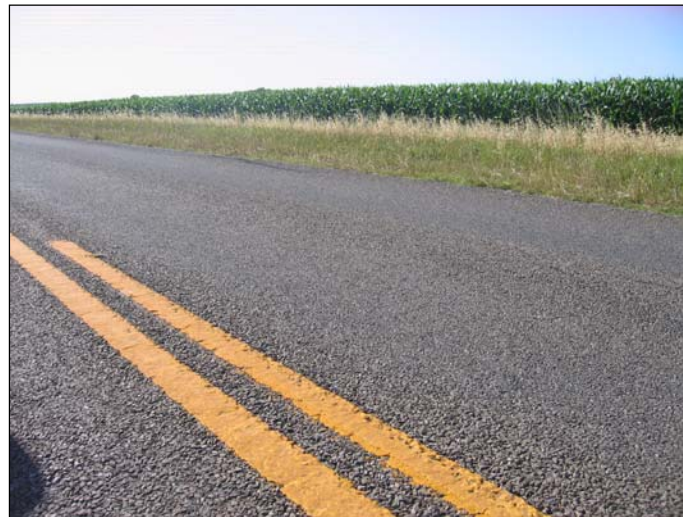
Figure 3.5. FM 487 Sampling Locations in Maintenance Location 8.
