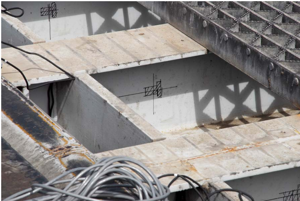
Figure 33. Photograph of Positioning Marks at Each Sensor Location prior to Grinding.
