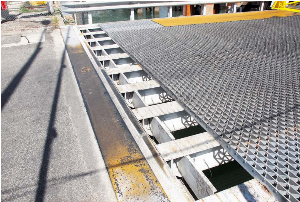
Figure 37. Photograph of Stringer Ends after All Sensors Installed.
