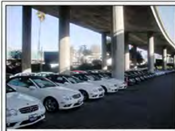
Parking Lot under a Viaduct in California Source: Caltrans Monthly Newsletter
