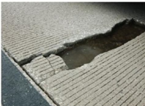
Punchout 1989-1990 Experimental sections (EB)
