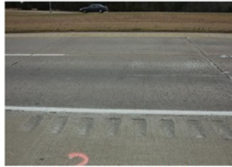
JCP slab in good condition
