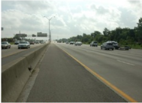
Beginning of survey, east of Calais St. 1989-1990 Experimental sections (EB)
