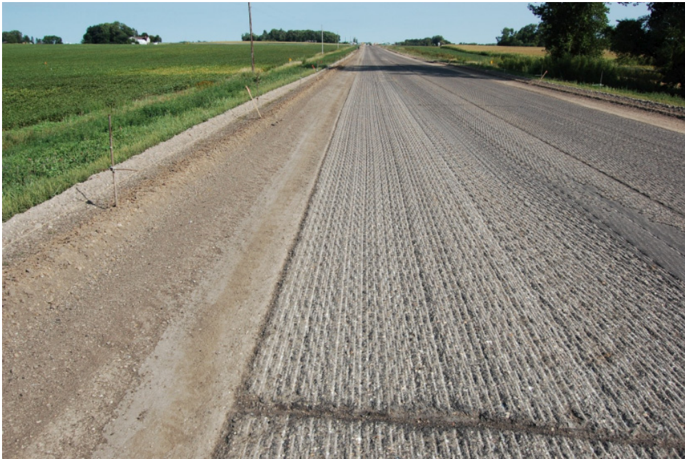
Figure 7.3: Milled existing asphalt pavement
