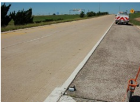
End of NB BCO at Holliday Creek bridge
