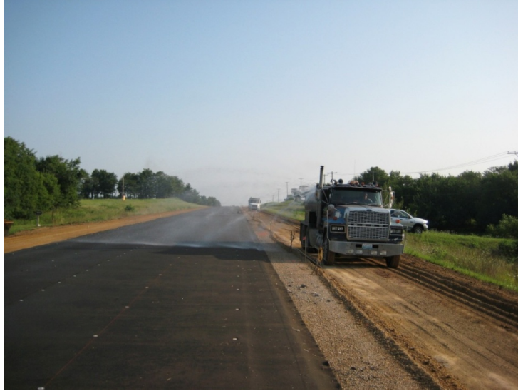
Figure 2.7: Cooling down the prepared surface before placement
