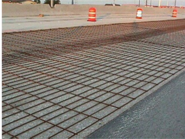
Figure 2.2: Steel placed directly on top of existing pavement
