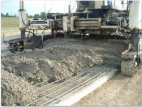
Ahead of the Paving Machine
