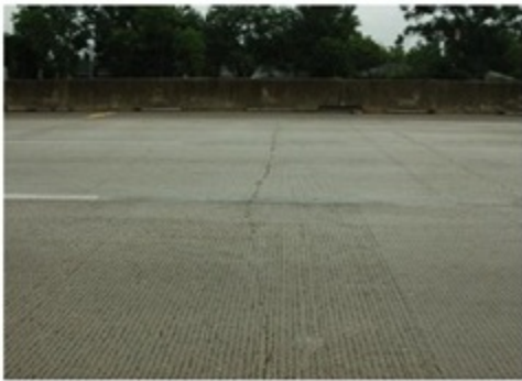
Transverse cracks
