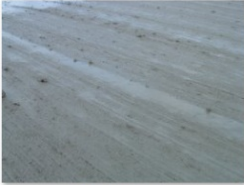
Finishing the Surface
