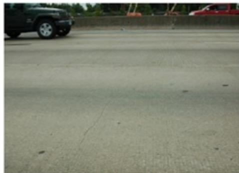
Transverse cracks
