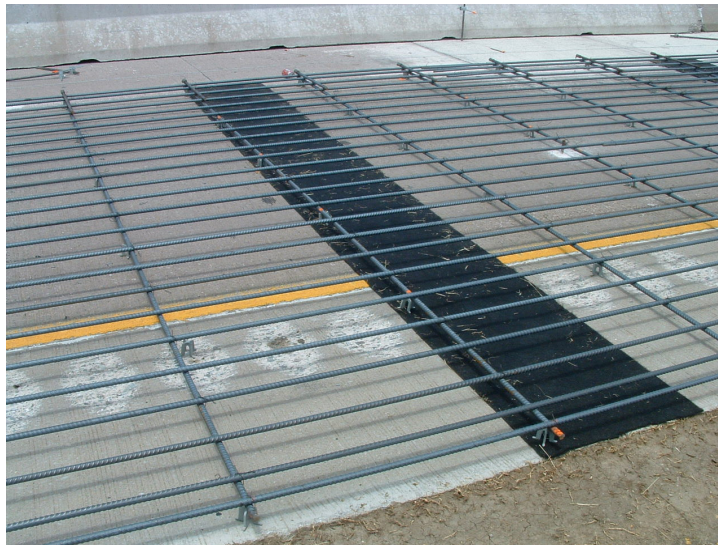
Figure 3.4: Prepared surface prior to the yellow stripe removal
