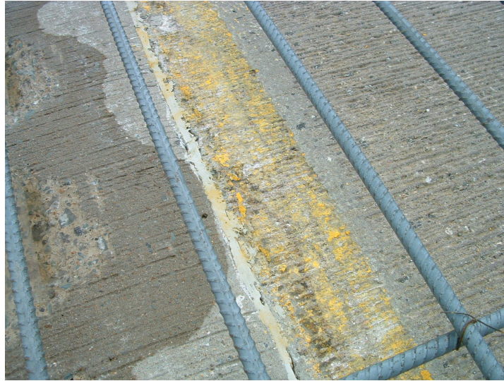
Figure 3.5: After the removal of the yellow stripe
