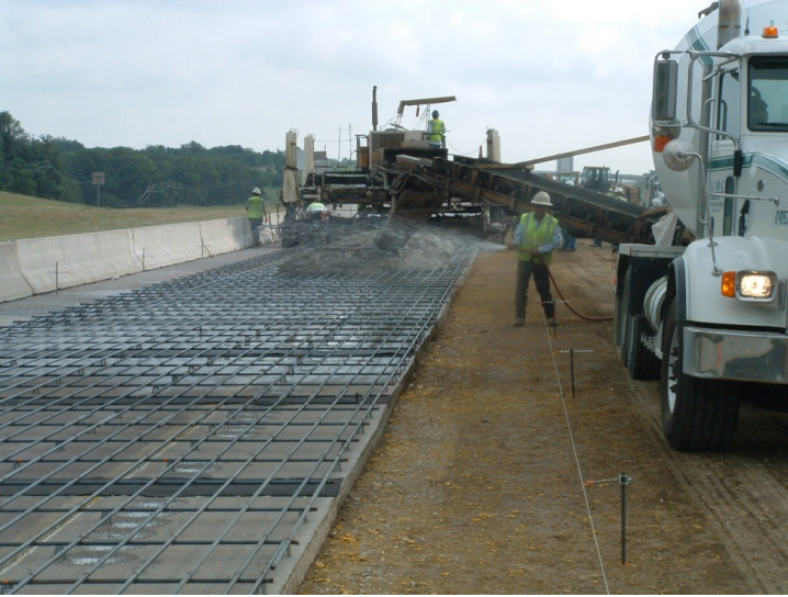
Figure 3.9: A worker spraying water on the surface ahead of the paver
