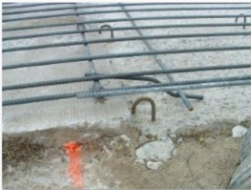
Reinforcement at Transition
