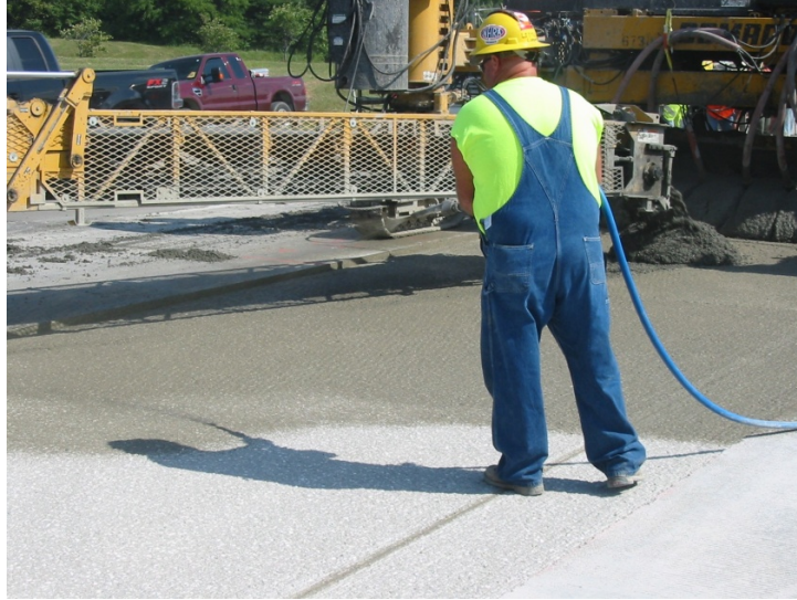
Figure 2.5: Spraying grout immediately ahead of paver
