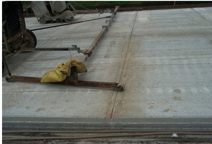
Figure 7.12: Early entry sawing
