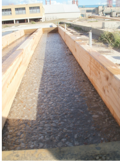
Figure 4.15: Exposed CA shown in the prepared surface in SSD condition
