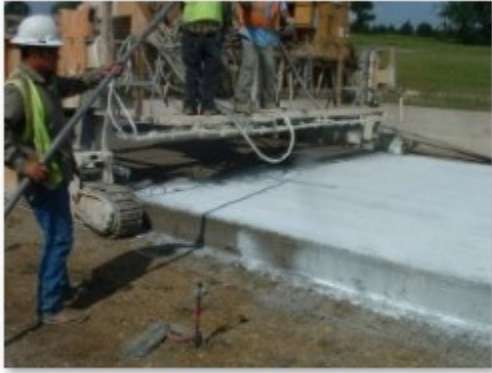
Spraying Curing Compound
