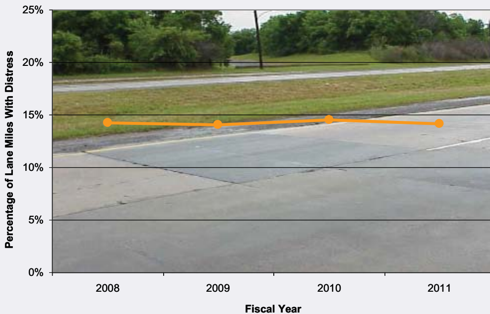
CRCP Concrete Patches (rated), FY 2008-2011
