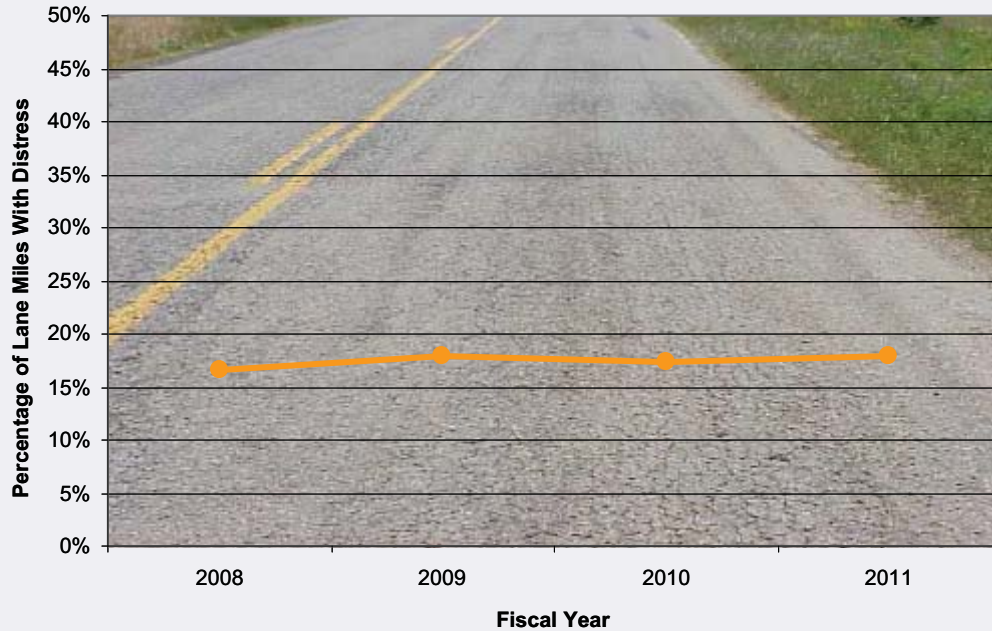
ACP Alligator Cracking (rated), FY 2008-2011
