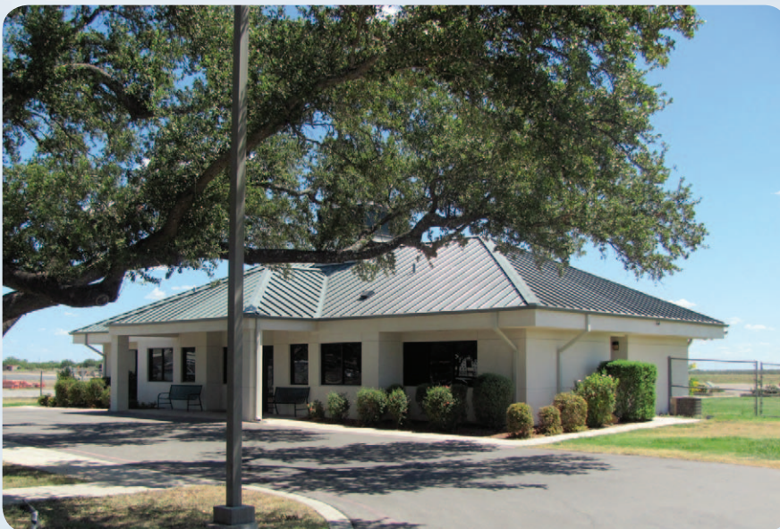
The terminal building at Garner Field Airport in Uvalde.
