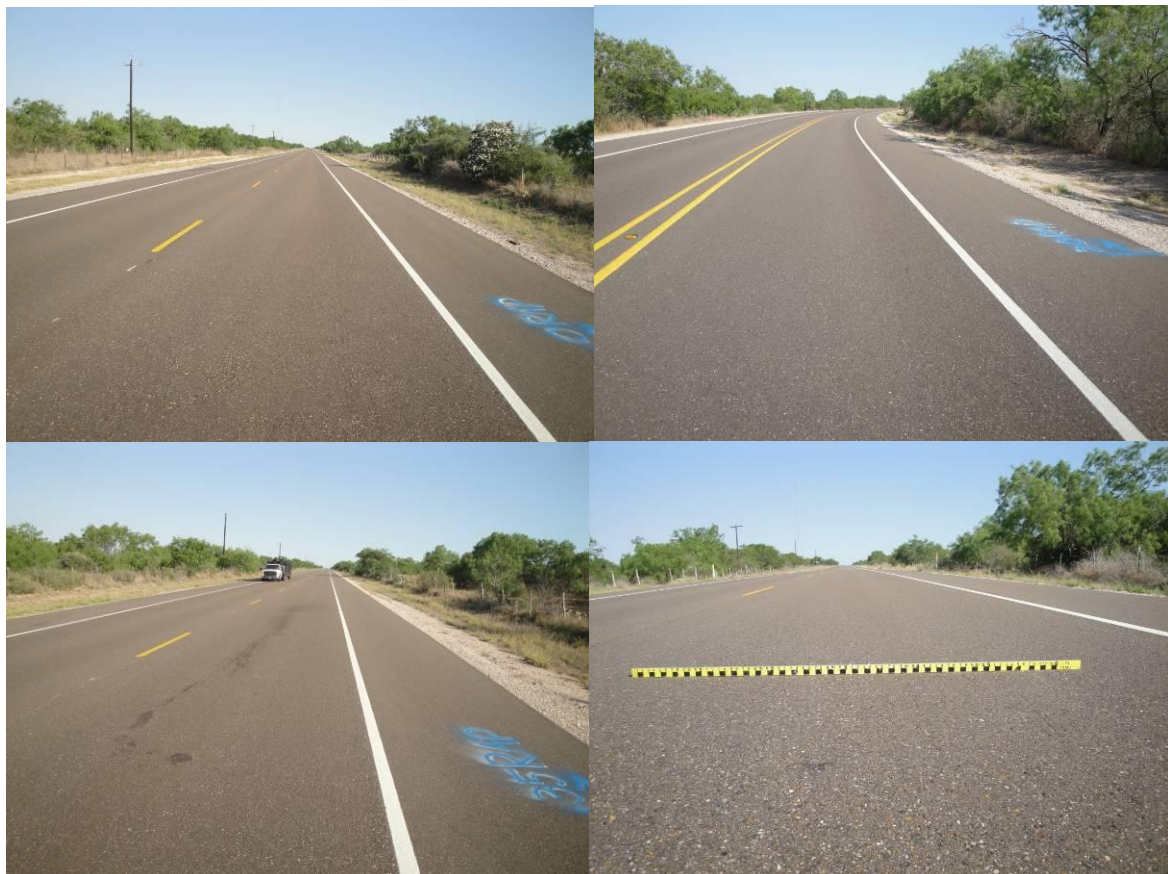
Figure 21. RAP Test Sections on FM1017: None of Rutting and Cracking on April 12, 2011.
