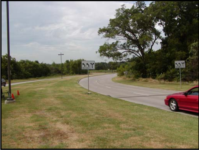
Figure 4-3. Advanced Traffic Sign – Southbound Gerault Road Approach.
