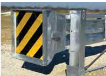
Familiar sight: the ET-2000 guardrail end treatment.
