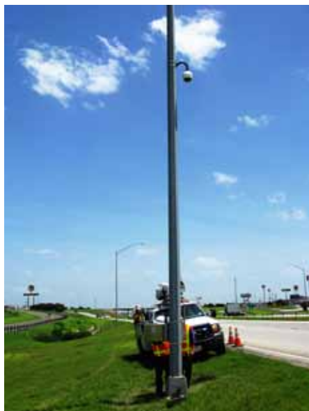
A travel-time monitoring station using TTI-developed software called AWAM is mounted on a light pole along I-45.
