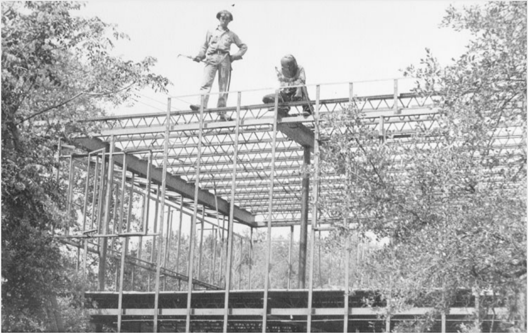
1938 construction pictures: welded steel frame
