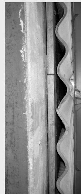
corrugated cement-asbestos panels
