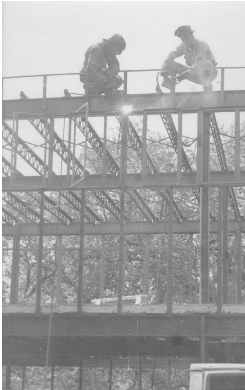
Figure 11 Perch construction Photo of welded steel frame
