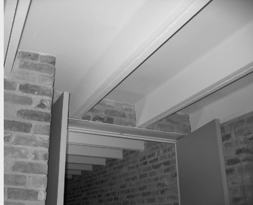
pre-cast concrete joists
