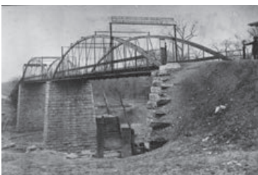
Toll bridge across the Trinity
