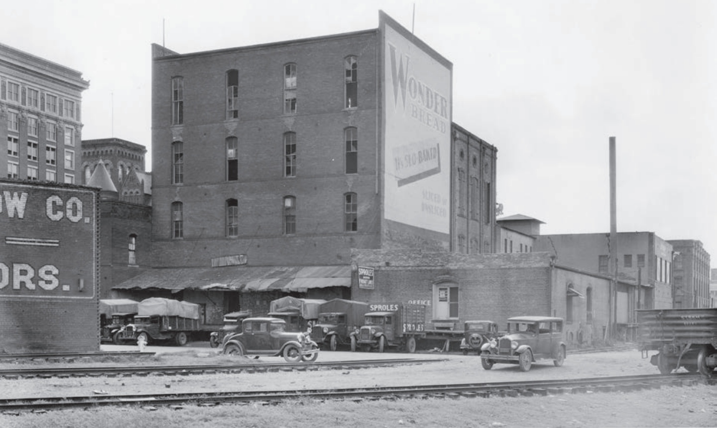
These buildings along Broadway, between Houston and the Trinity River, were demolished beginning in 1934 to make way for Dealey Plaza.
