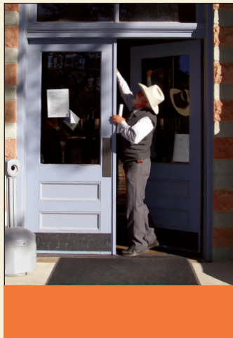
Ongoing maintenance at Jeff Davis County Courthouse.
