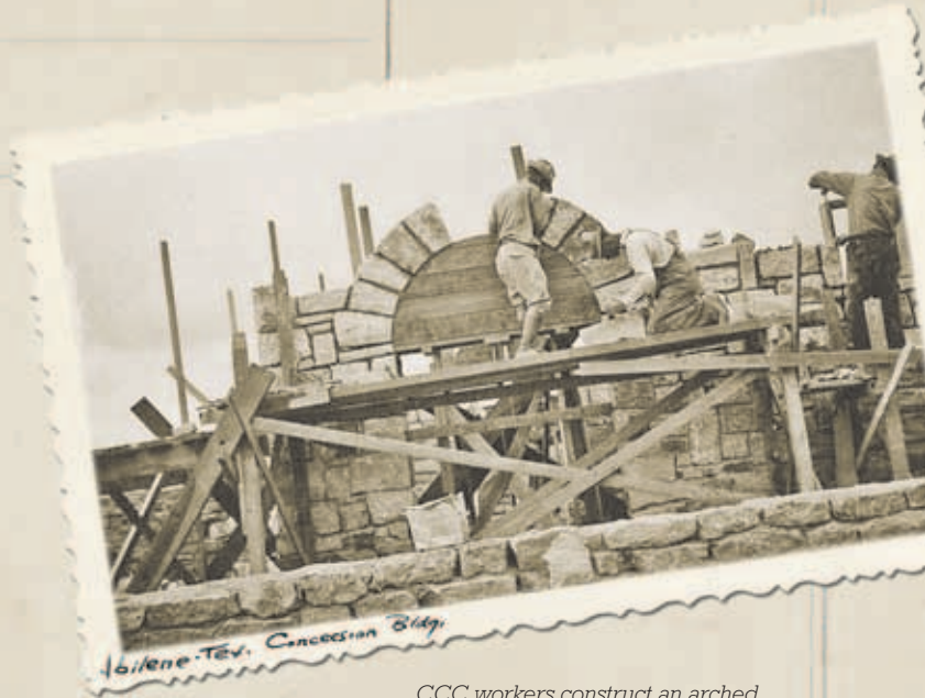
CCC workers construct an arched opening at the concession building.
