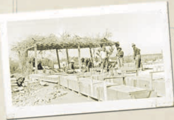
The men of Company 886 built forms and combined the locally plentiful lime-rich caliche soil with cement and then cast caliche crete blocks. Nearby stands a brush-covered ramada, typical South Texas shelter, which will protect the curing blocks.
