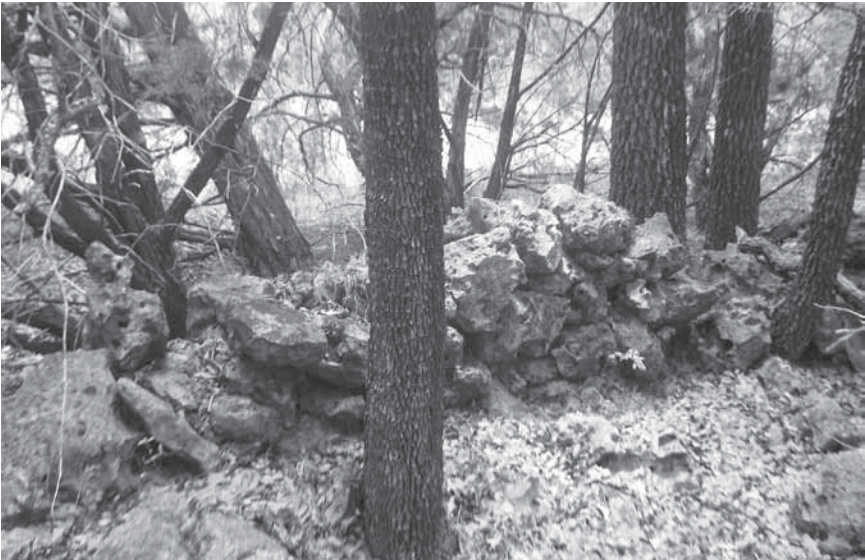
Figure 4. One of the rock walls on the A.C. Hughes tract, which probably enclosed the field where Trammell and Jones raised their crops. Photo 2010 by author.
