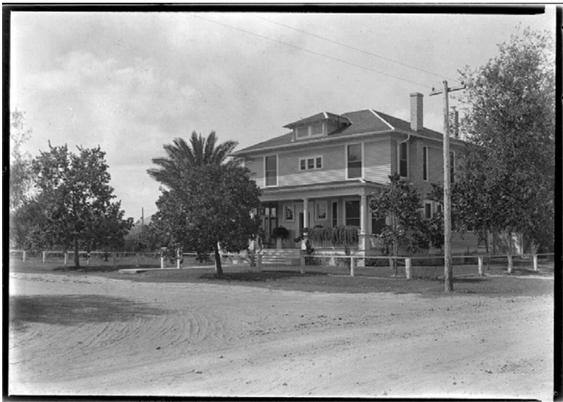
North East view of West Washington home.
