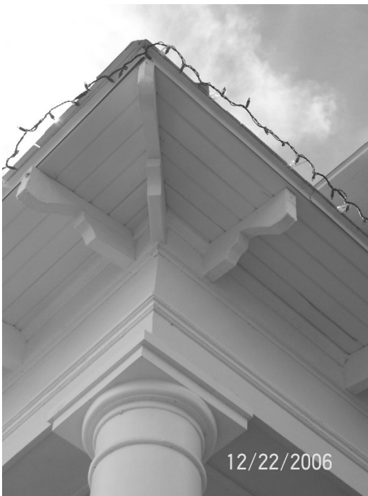
Image of the decorative brace and Tuscan style column.
