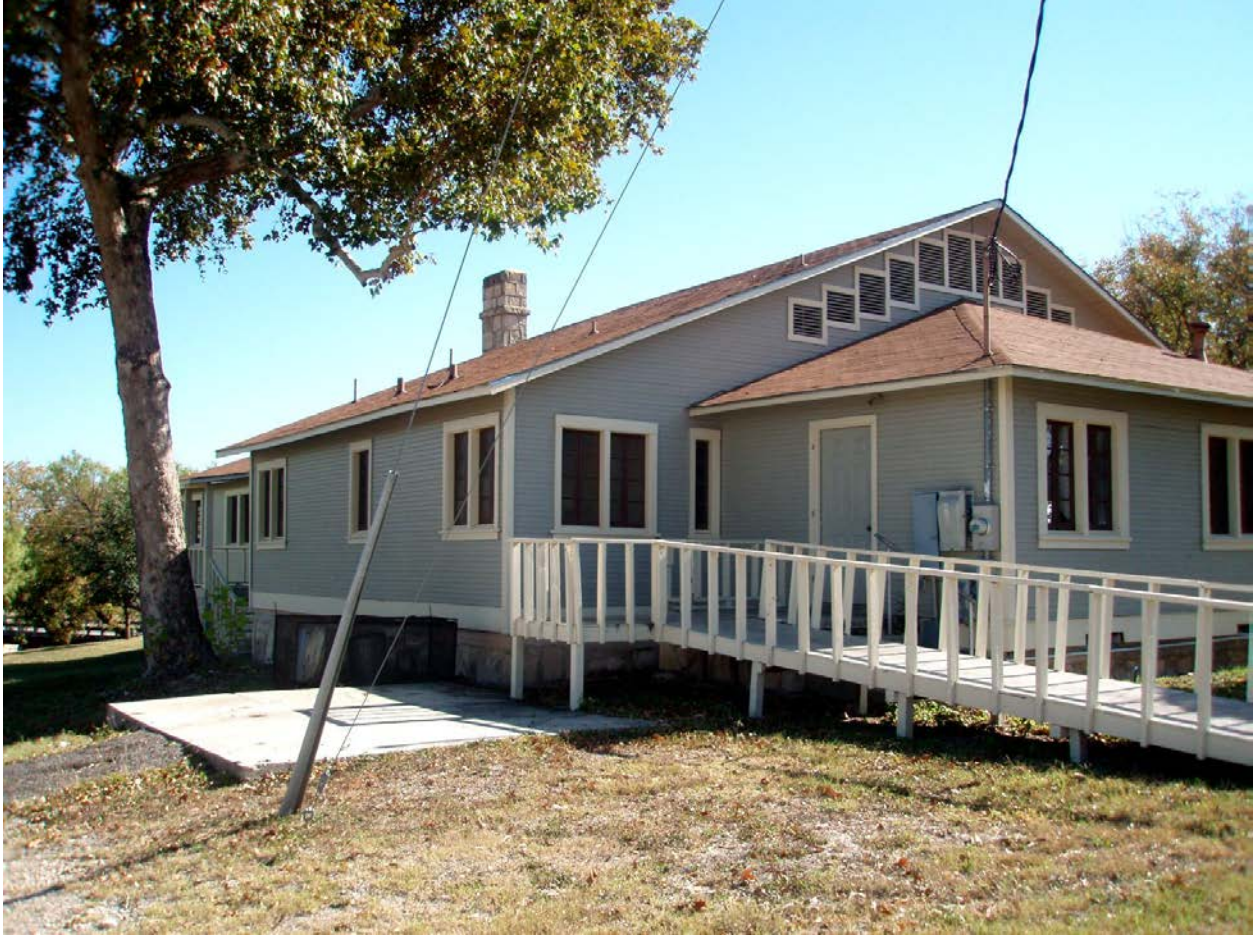
U.S. Army Service Club, Fort Clark, Texas back corner [West] elevation.
