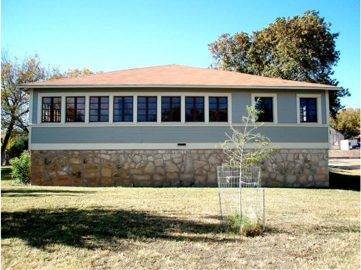
U.S. Army Service Club, Fort Clark, Texas side [Northeast] elevation.
