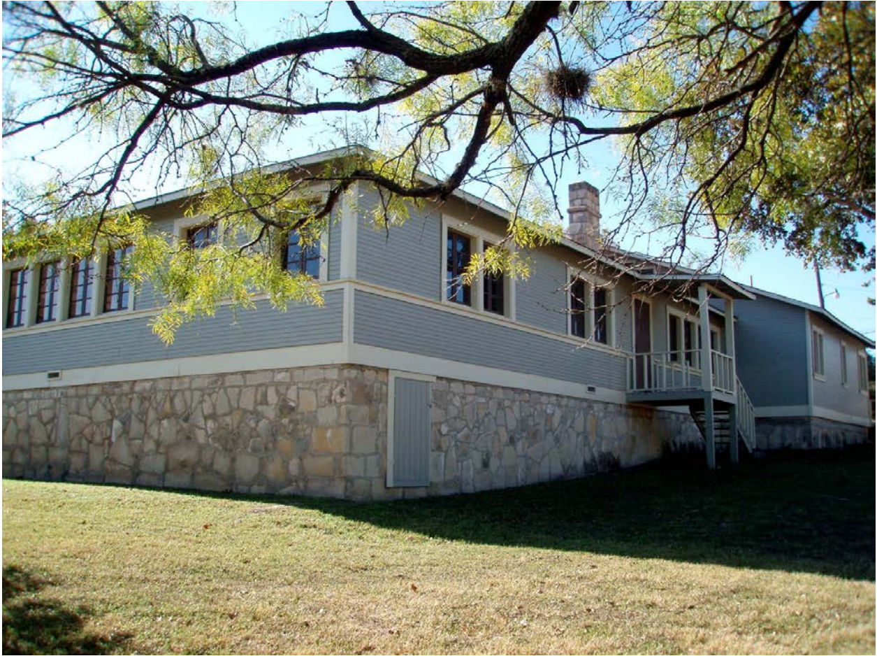
U.S. Army Service Club, Fort Clark, Texas back corner [North] elevation.
