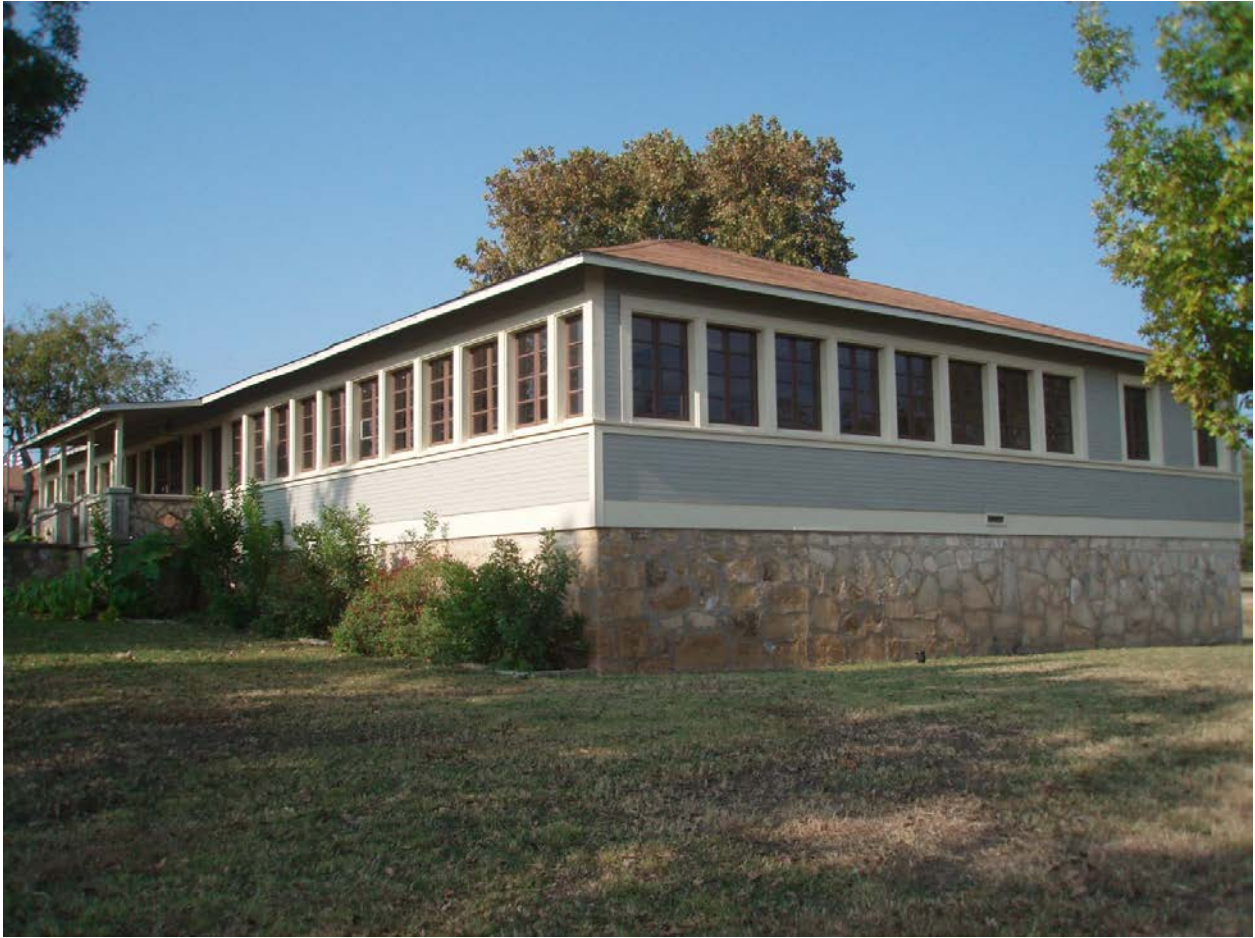
U.S. Army Service Club, Fort Clark, Texas front corner [East] elevation.
