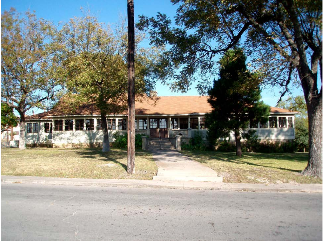
U.S. Army Service Club, Fort Clark, Texas front [Southeast] elevation.
