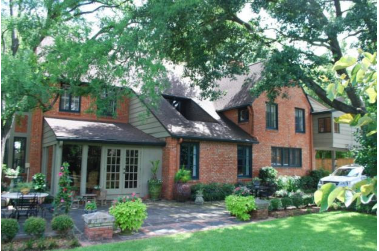
Oblique of east and north elevations, view south
