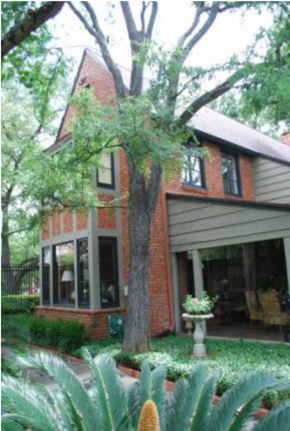
East elevation, view south Anna Mod for SWCA, 2010
