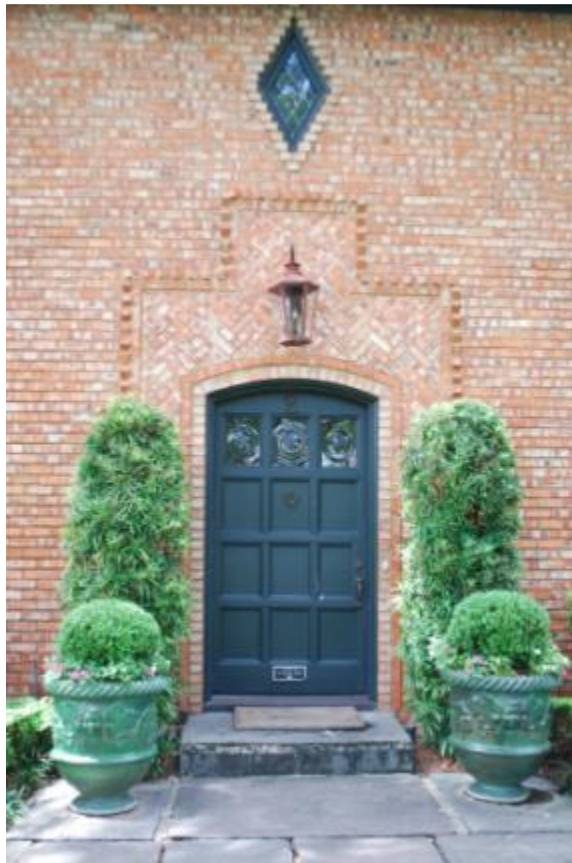
Front door detail
