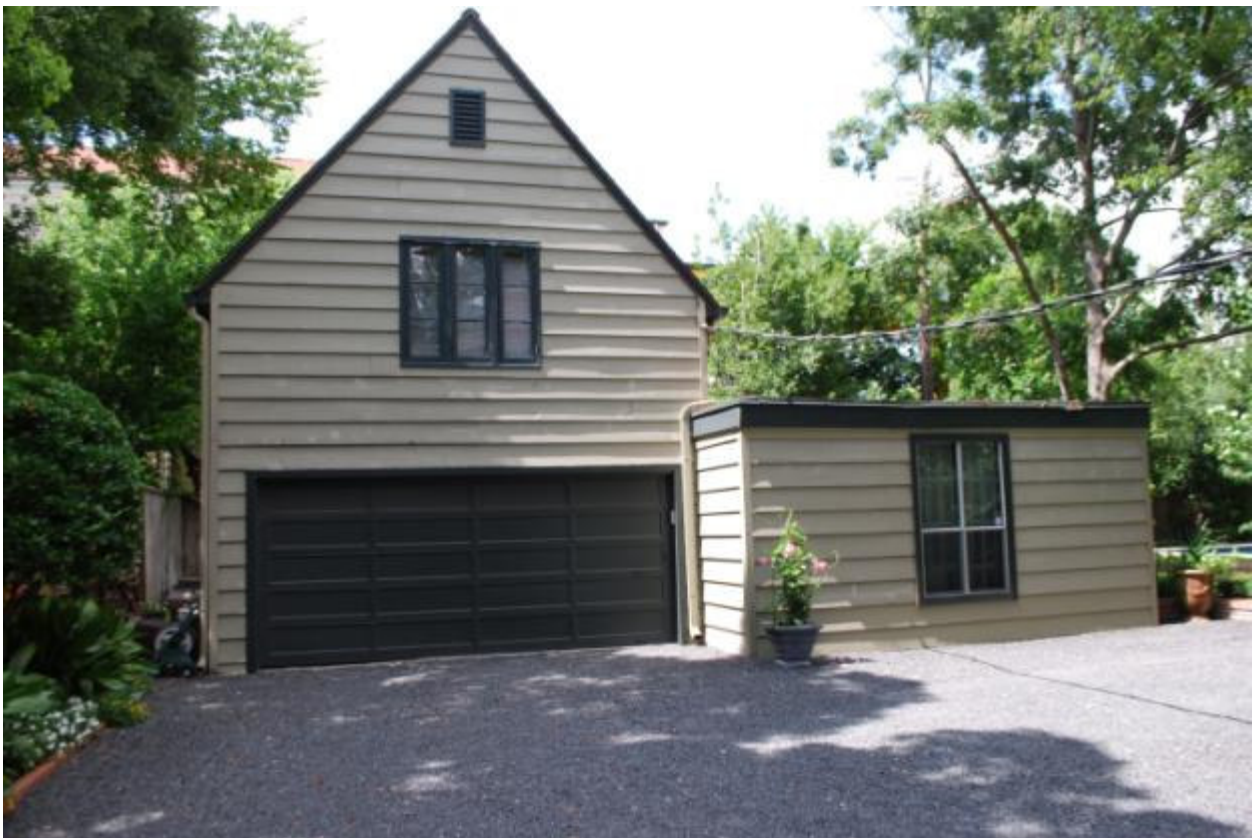
Garage and garden shed addition, view north
