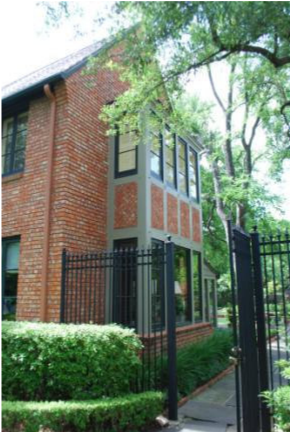
East elevation, view north
