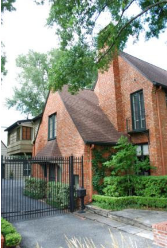
West elevation, view north
