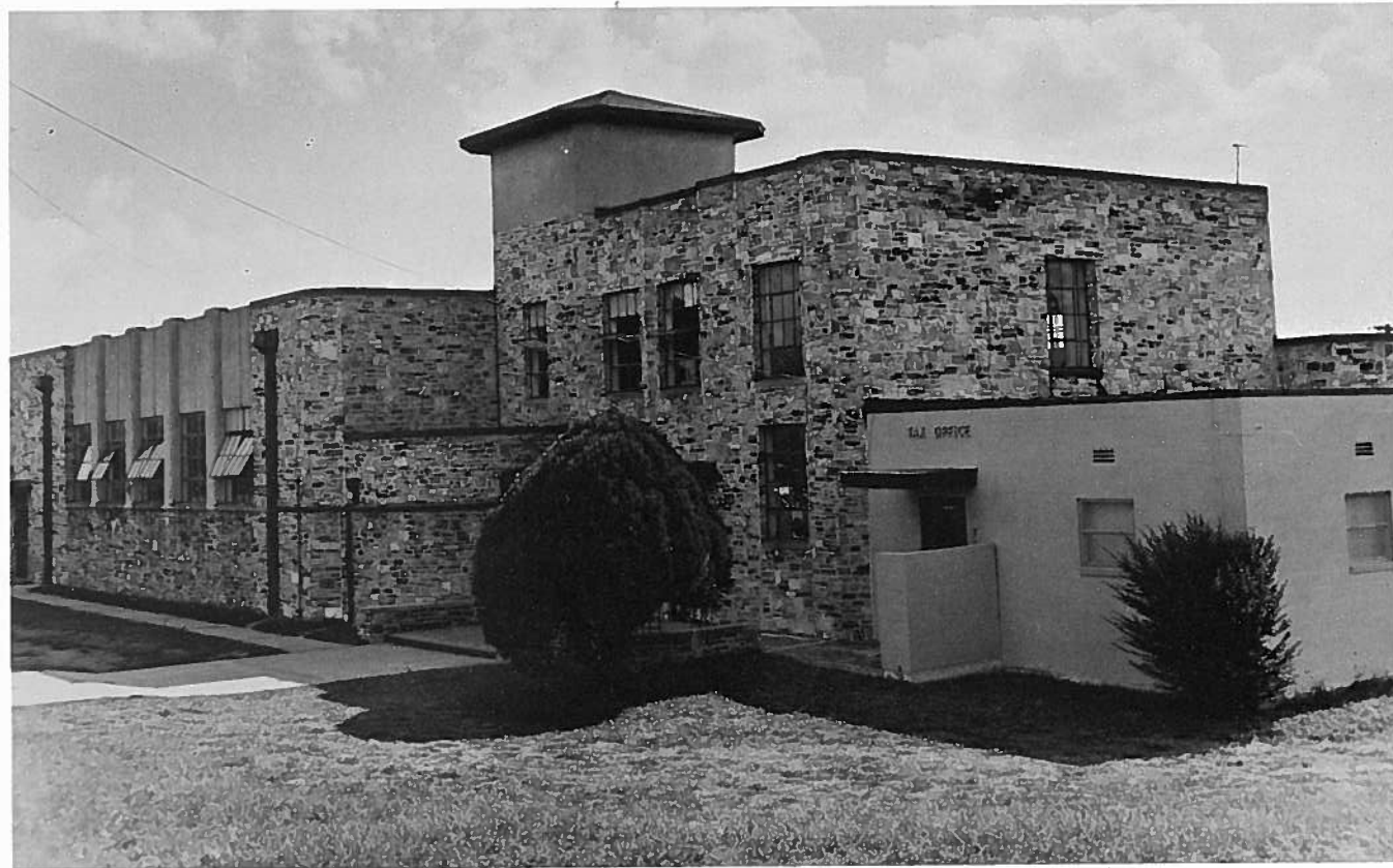
Mr. Will Weeren was the contractor of this school which was built 1938-40.
