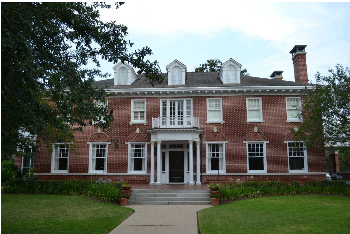
#25 Courtlandt Place, north façade, view south
