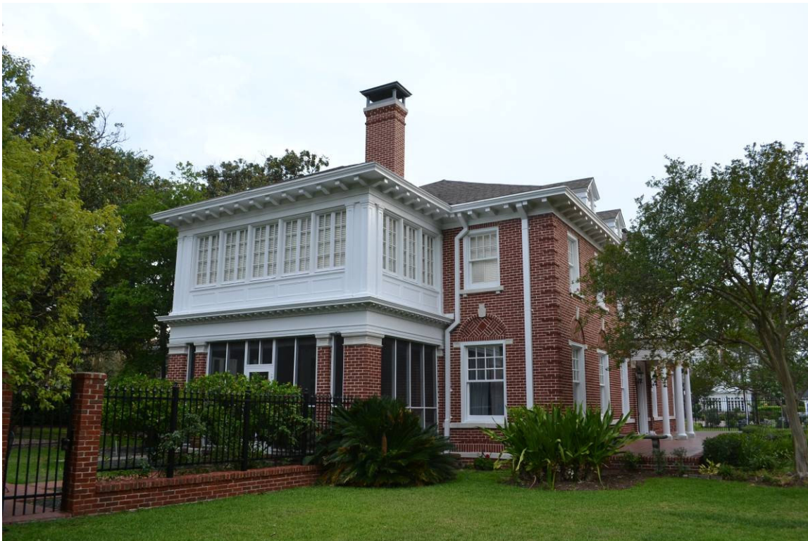
East elevation, view southwest
