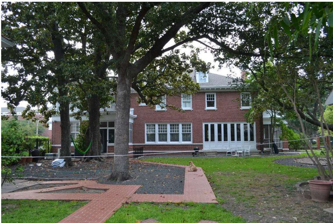
South façade, view north
