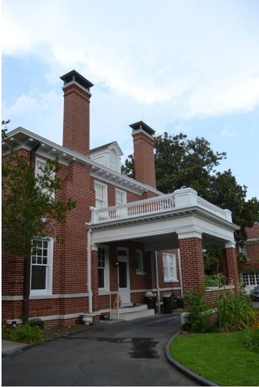
West elevation, view south Grace Cynkar for SWCA 2011
