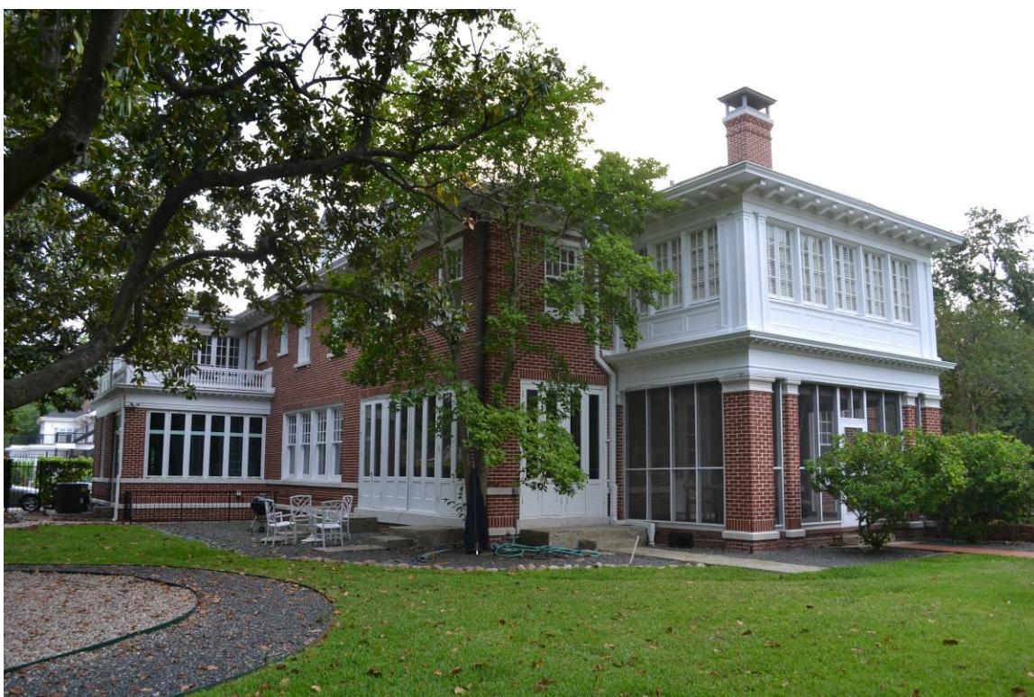
Oblique of east and south elevations, view northwest
