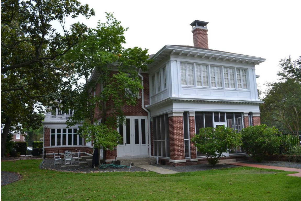
East elevation, view west
