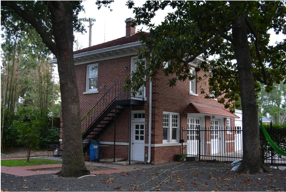
Oblique of garage east and north elevations, view southwest
