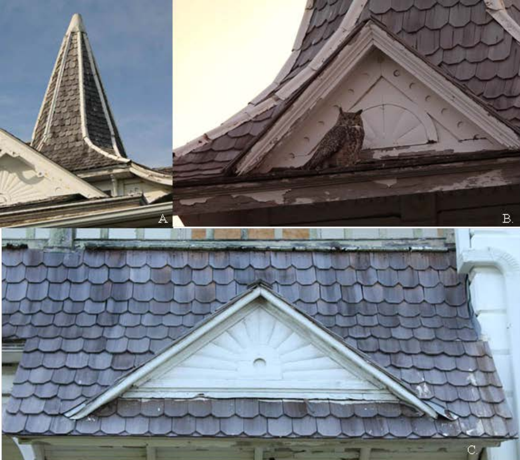
Fig 24. Shingle design on (a) spire, (b) base of spire and (c) over the front steps.
