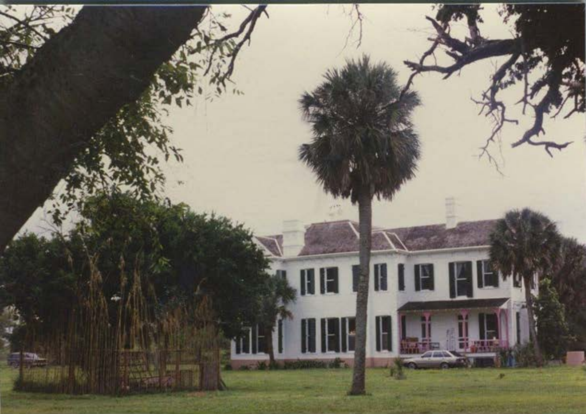
Fig 12. Archival picture of the north elevation showing the universal use of storm shutters.
