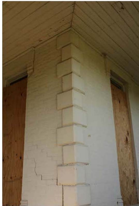
Fig 15. Brickwork and quoins
