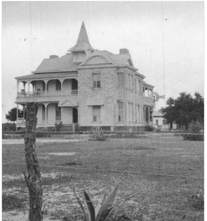
Fig 9. Early 20th Century Photograph of the Rabb House. Note: the second floor rear porch and windmill are now missing.
