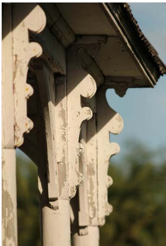
Fig 18. Detail of second floor porch post brackets.
