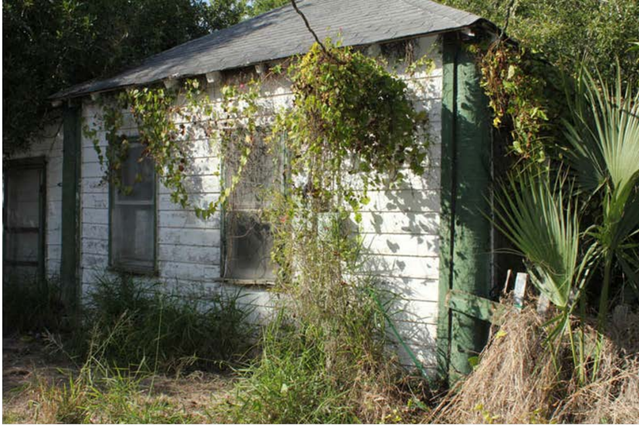
Fig 7. Palm log house thought to be the foreman's house.
