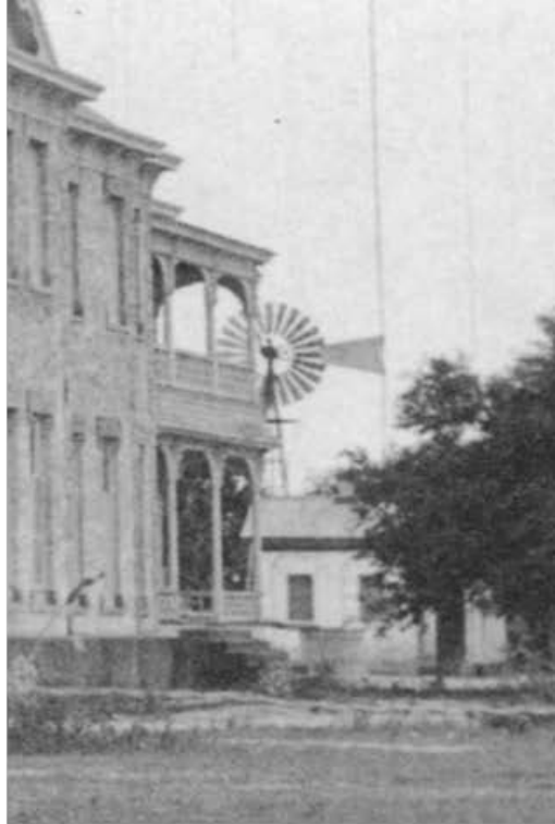
Fig 38. Close-up photo showing that at one time house had a second floor covered porch on northwest corner.
