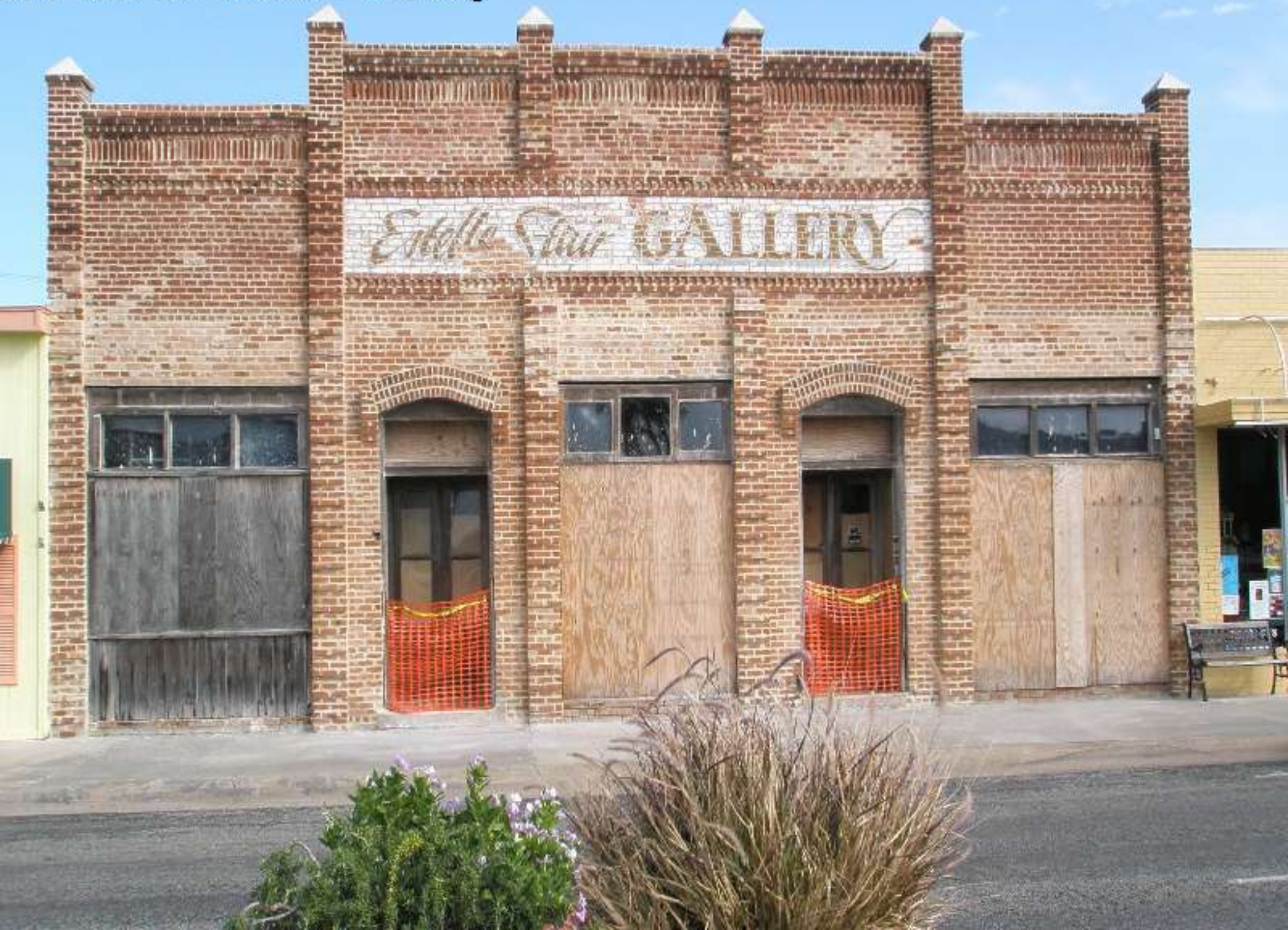
2007 front view Sorenson Stair bldg
